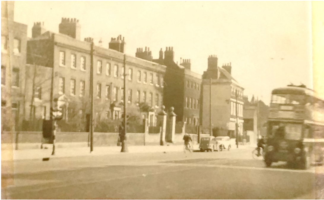
Figure 11 - May 1939 of 790-800 High Road. Number 792 projects forward, covered in ivy. Nos. 794 and 798 are symmetrical, each side of Percy House.
