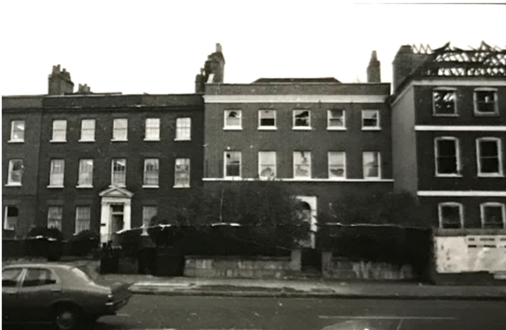
Figure 14 – Numbers 790 to 794 after the fire.
