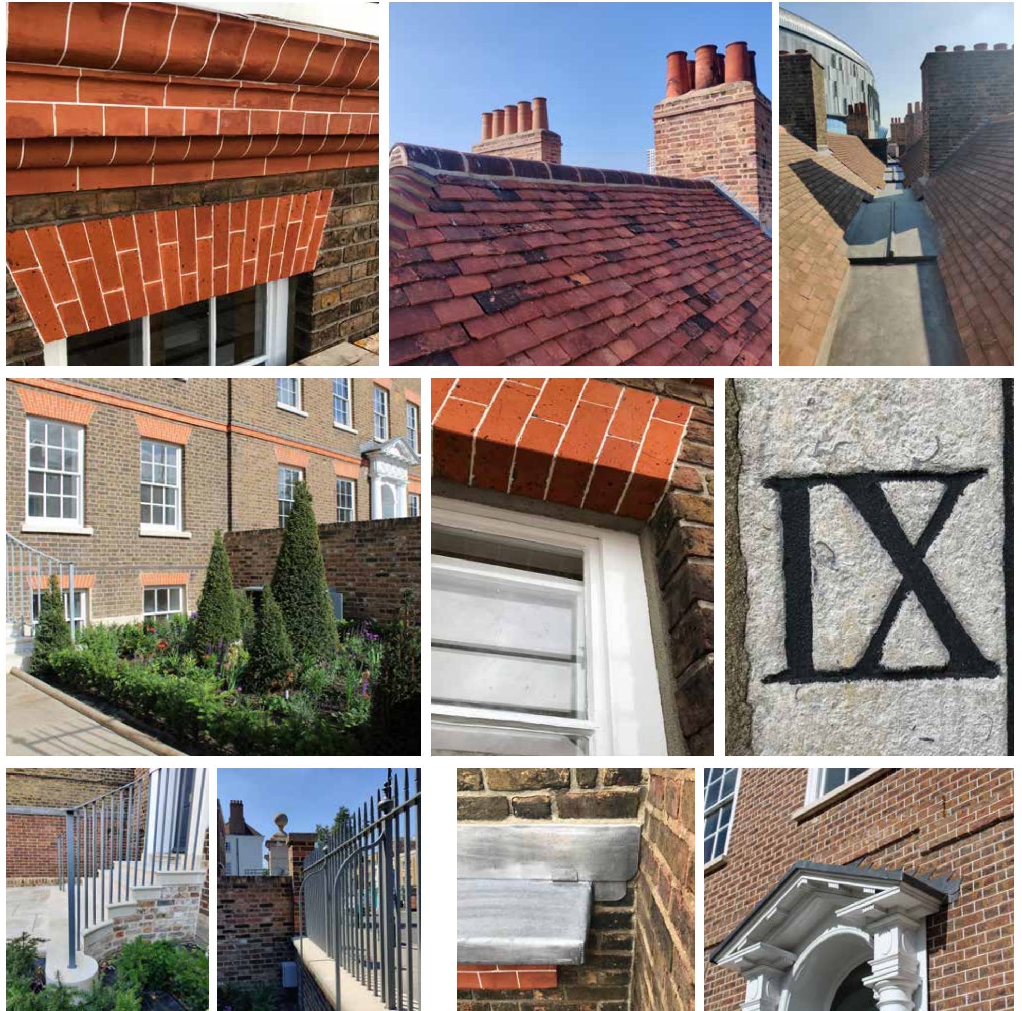
FIGURE 14. - Northumberland Terrace Post Restoration
