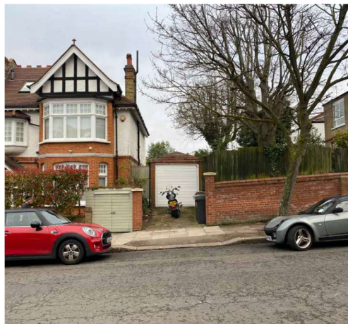
Photo 2 - The garage with existing narrow access
