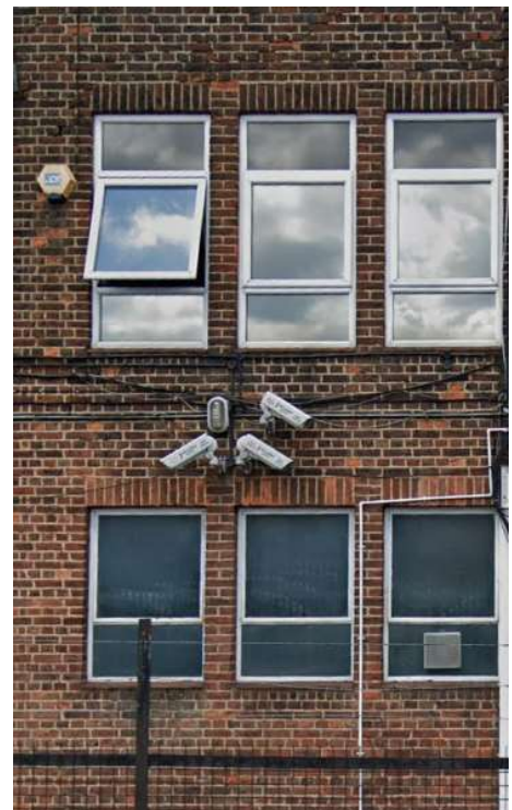
Existing Roeder House
