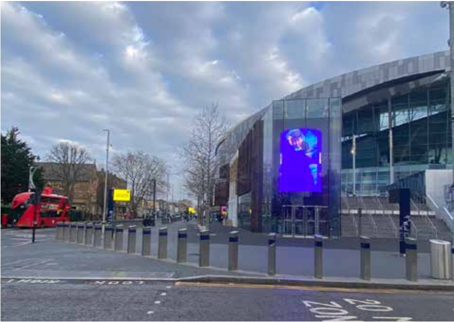
Existing view of the Stadium and High Road from Park Lane
