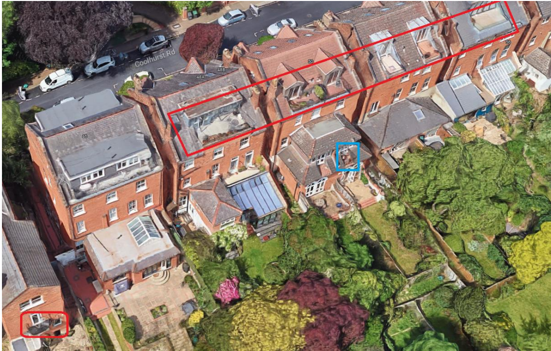
Balustrades on the host building (blue) and adjoining properties, which form part of the local character
