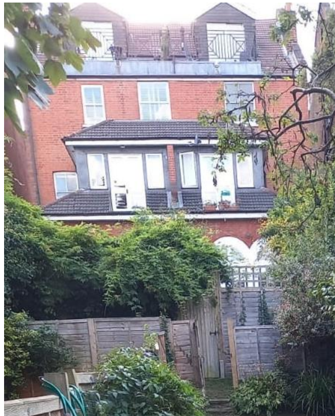
An old photograph showing a chair on the first floor balcony
