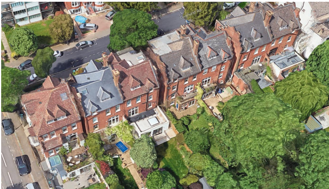
Various balconies and diverse rear elevation of other properties in Coolhurst Road
