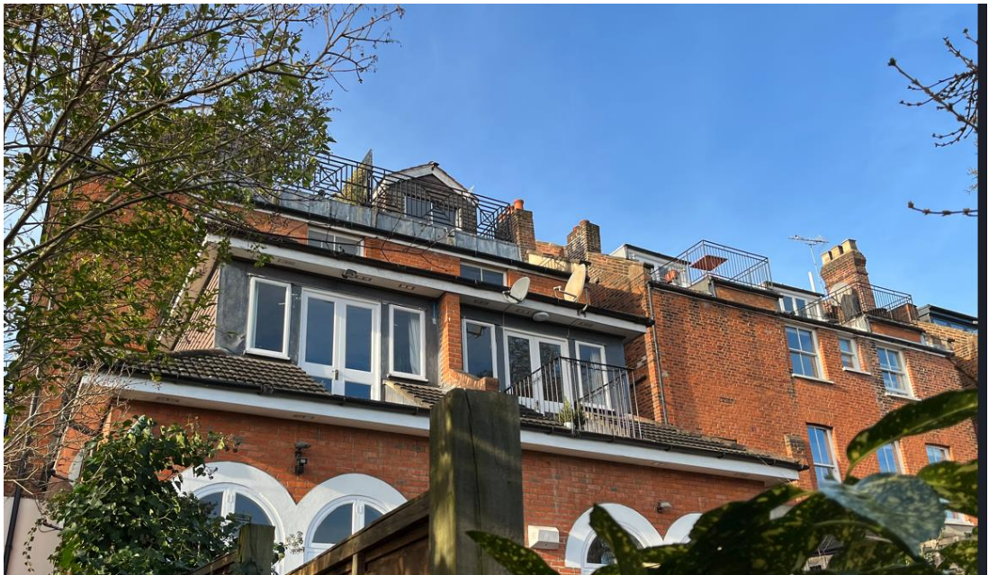
Various existing balconies and windows that result in a degree of mutual overlooking
