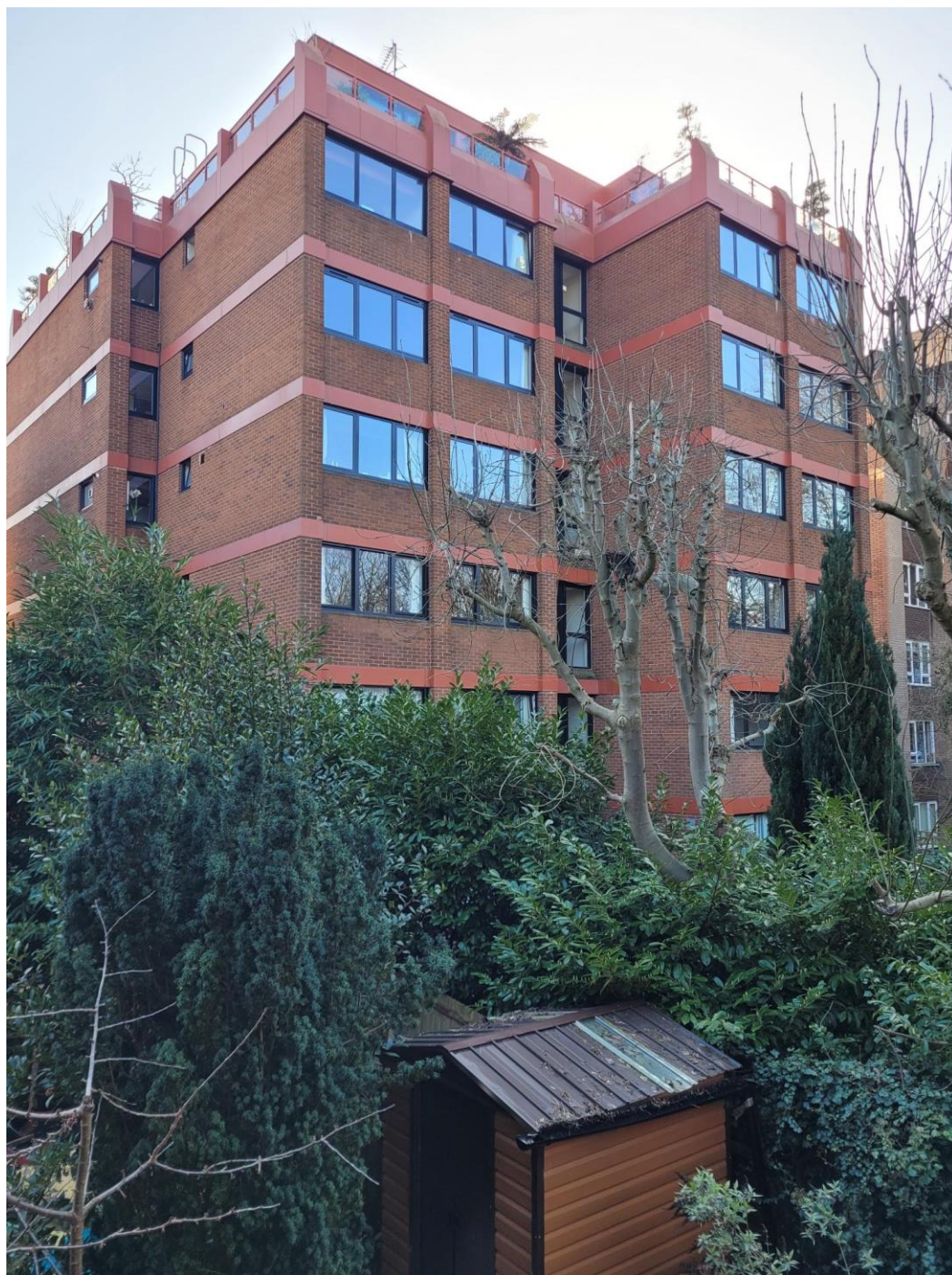
View of 125 Hornsey Lane from 6 Colwick first floor window
