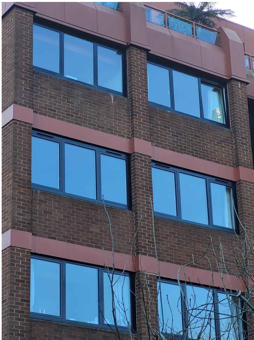
Lifesize view of upper flats
