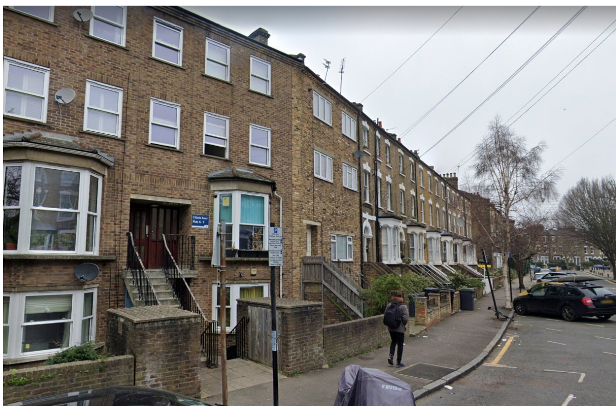
Application site (centre) looking north
