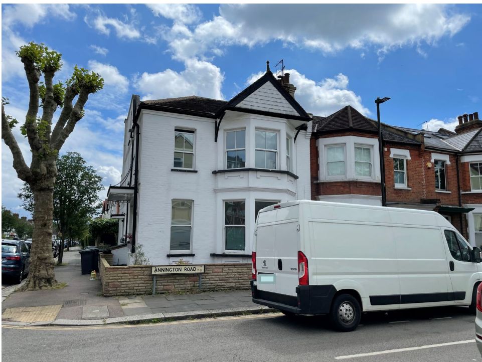
View of the front elevation
