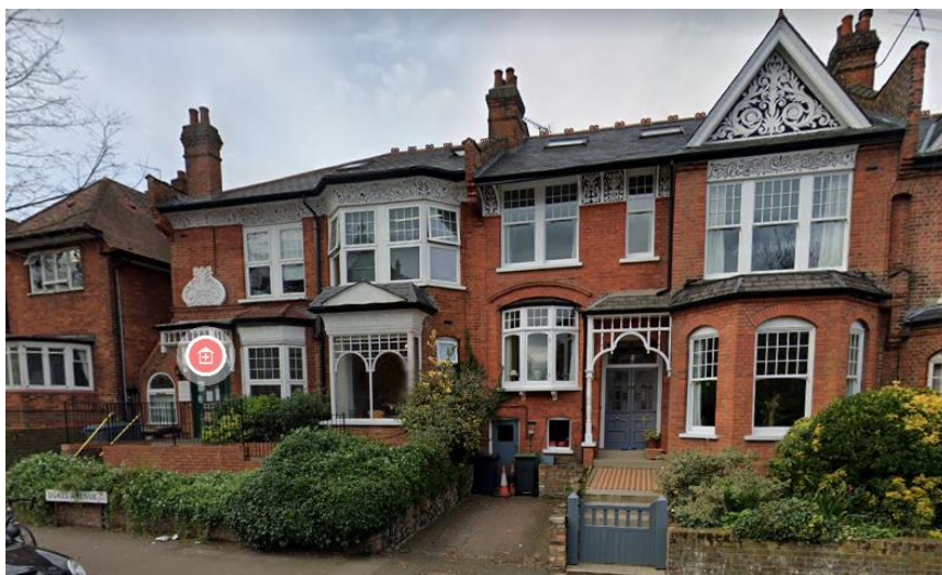
Figure 7. Photograph of existing secondary door to no.3 Dukes Avenue
