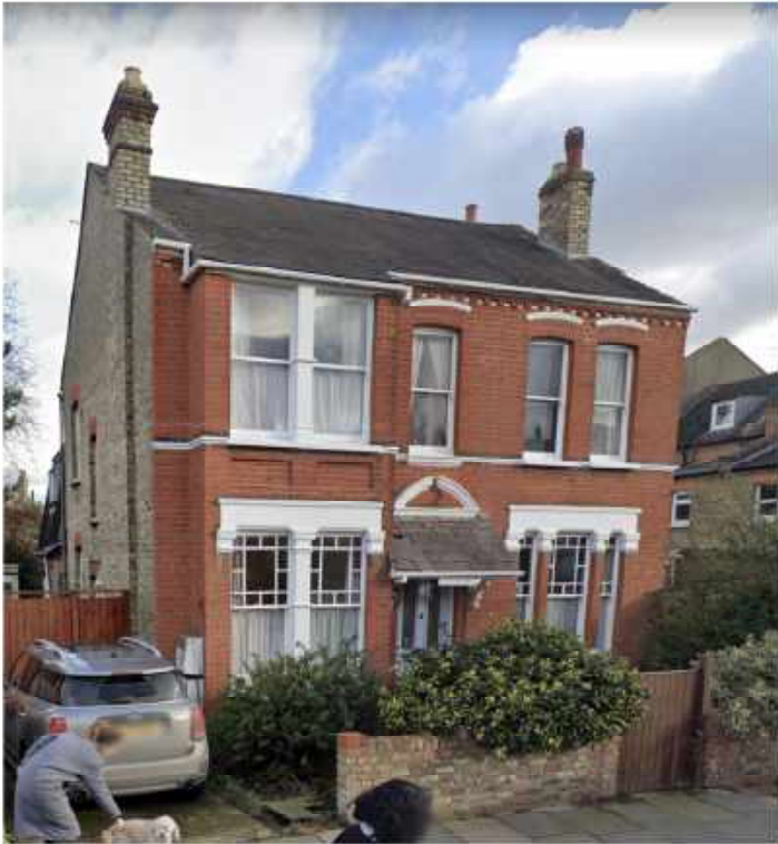
Photograph of front elevation of main building
