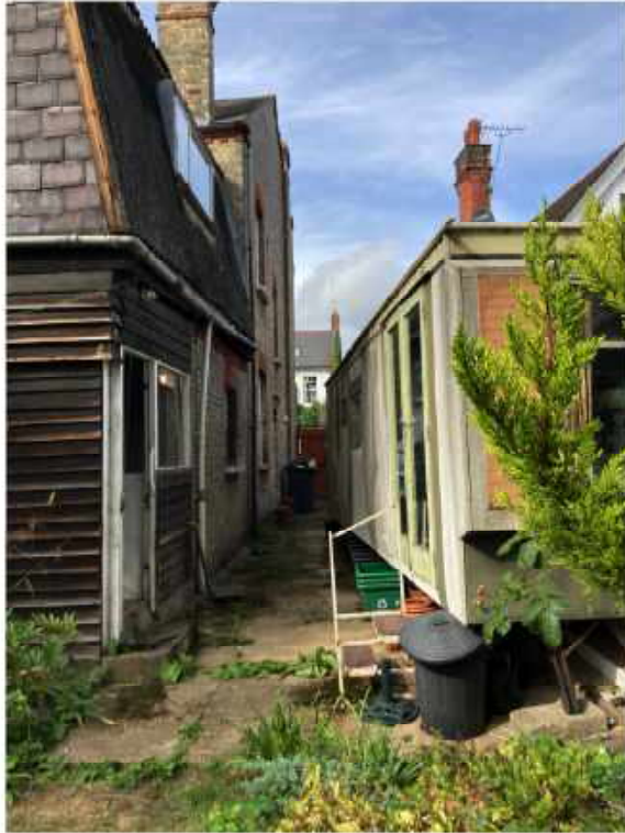
Photograph of rear closet wing, north facing flank wall of main building and single story prefabricated building
