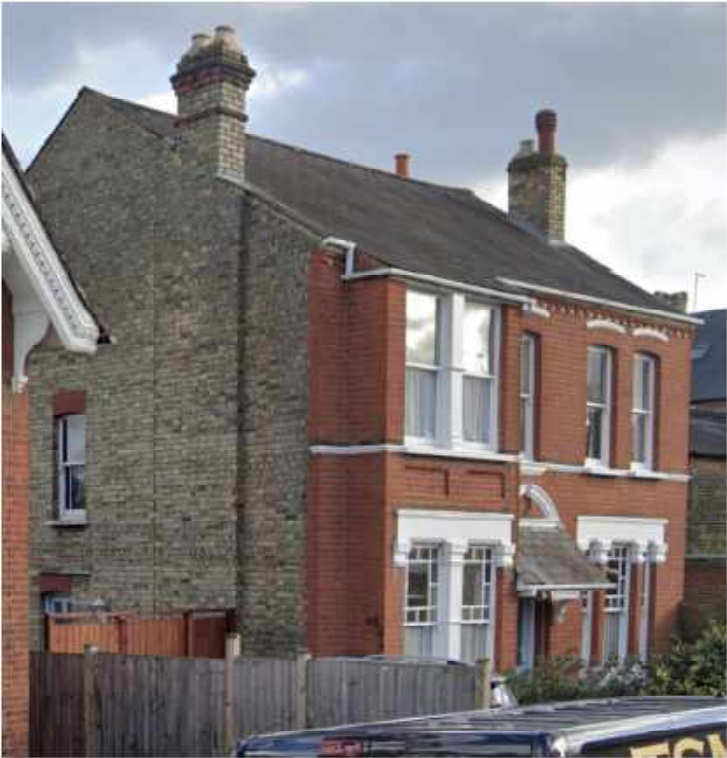
Photograph of north facing flank wall and front elevation of main building
