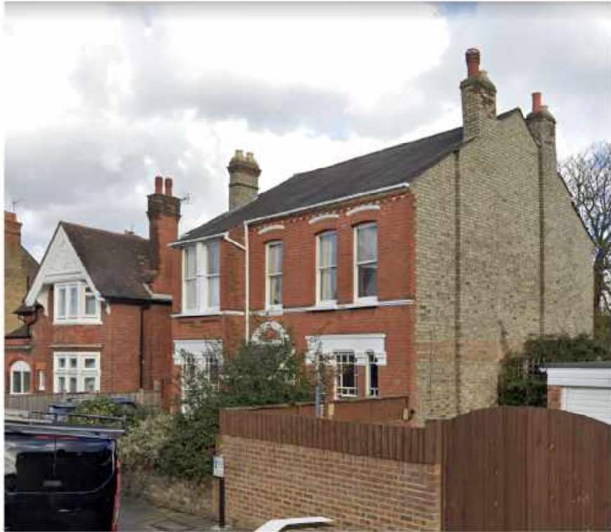
Photograph of south facing flank wall and front elevation of main building
