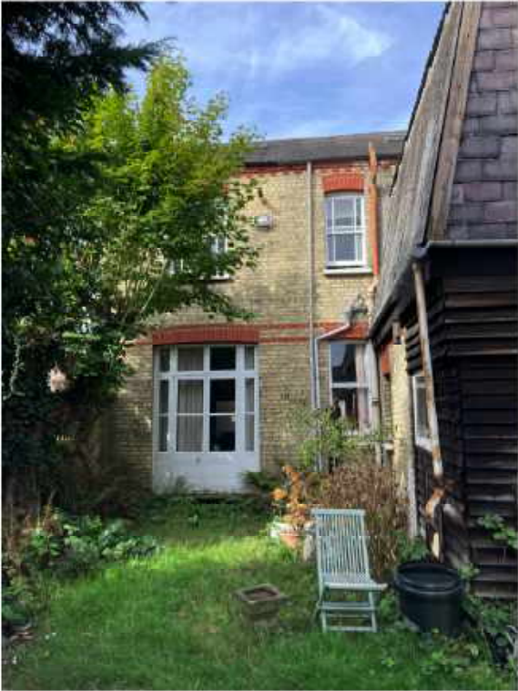
Photograph of rear elevation of main building
