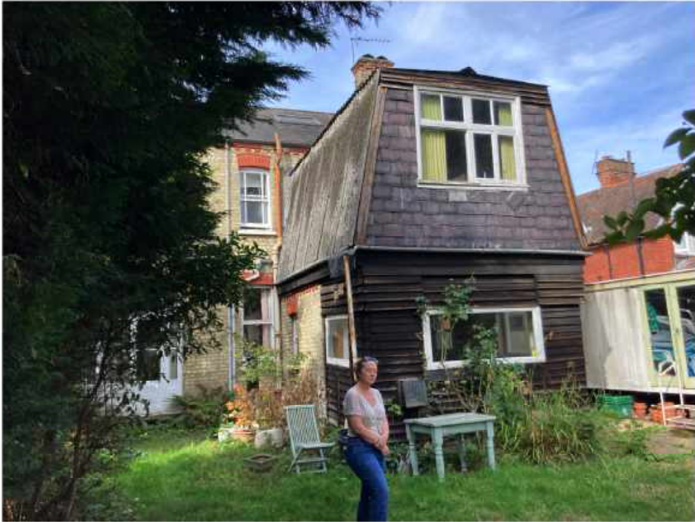
Photograph of rear elevation of main building and rear closet wing
