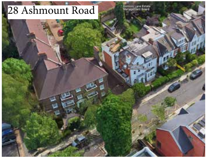
Image no.9: view end-of-terrace roof terrace
