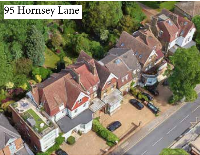
Image no.8: view end-of-terrace roof terrace
