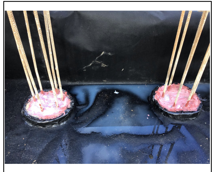
Overview of sealed pile heads
