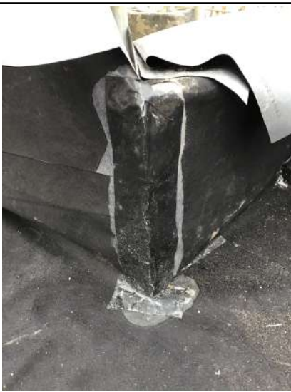
Corner detailing completed.
