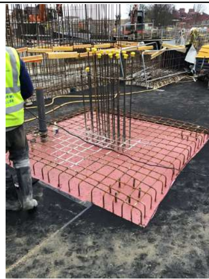
Large pile cap sealed.
