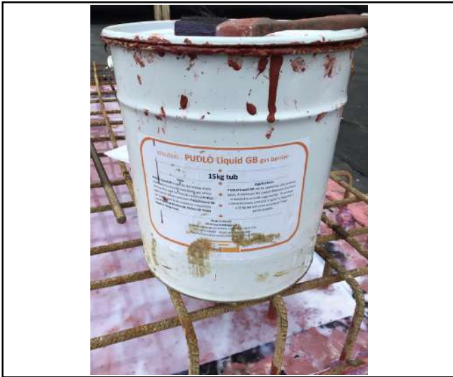
Pudlo liquid gas barrier applied to all pile caps.
