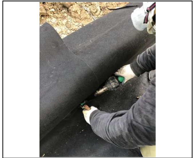
Installer welding a lap joint using hot air leister and roller.
