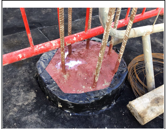
Pile heads fully sealed
