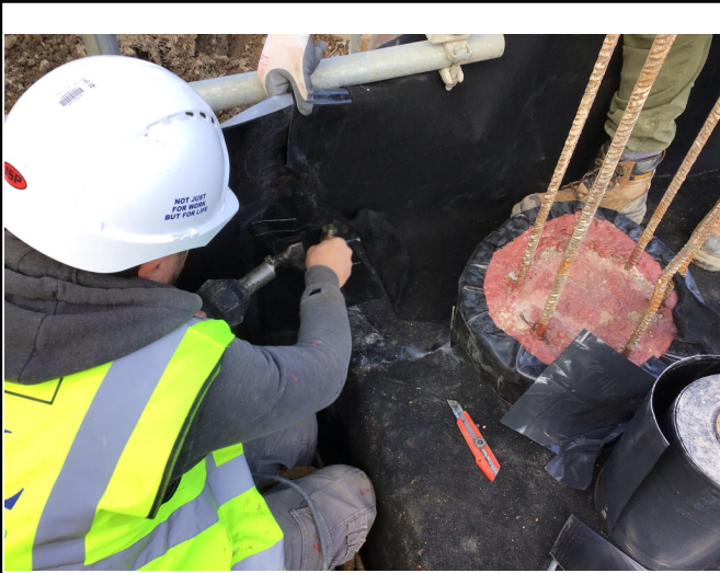
Last section of installation witnessed
