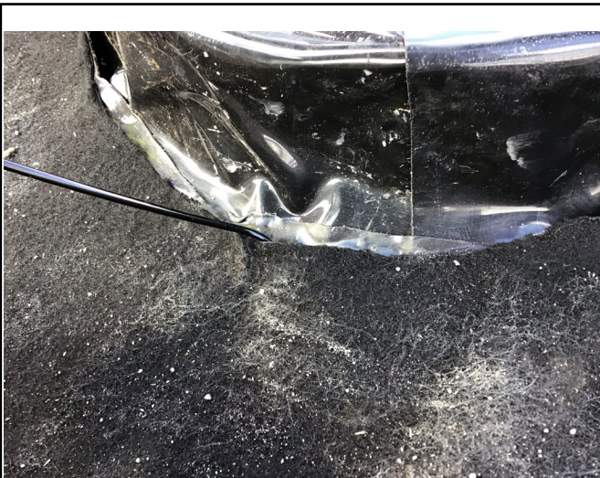
Pile heads fully sealed to Pudlo
