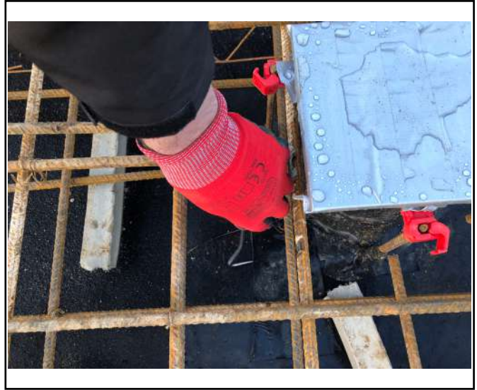
Pick and probe test to penetrations through steel.
