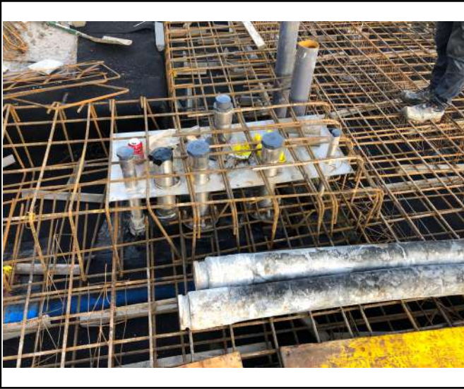
Penetrations from last visit have now been sealed.
