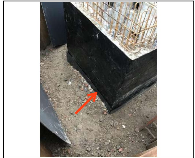
Protection board installed around
