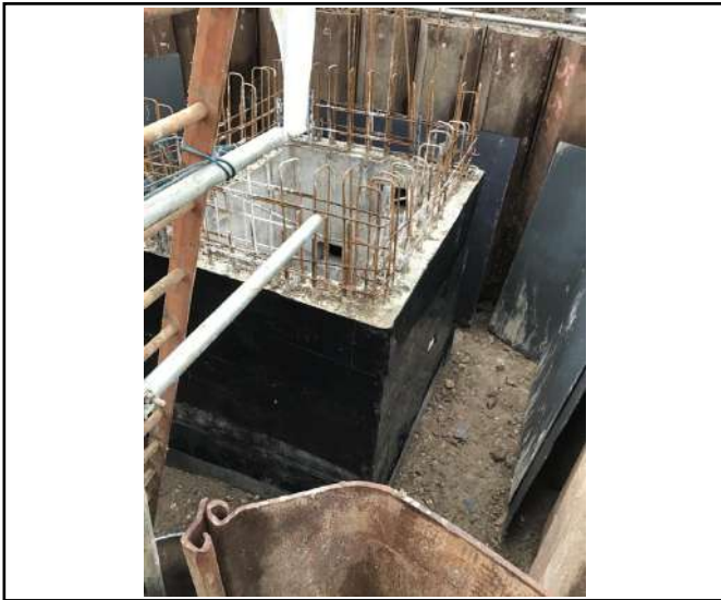
Protection board ready to be installed.
