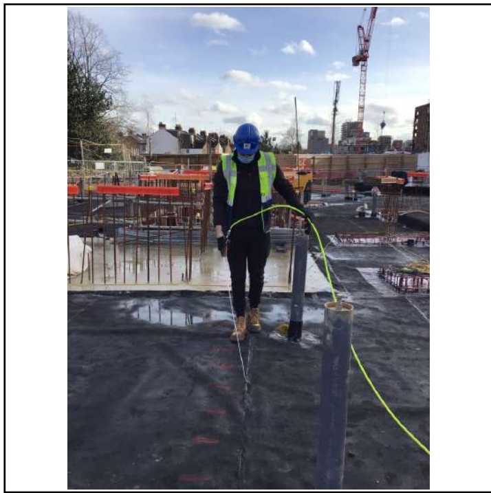
Air lance integrity test being carried out to welds.
