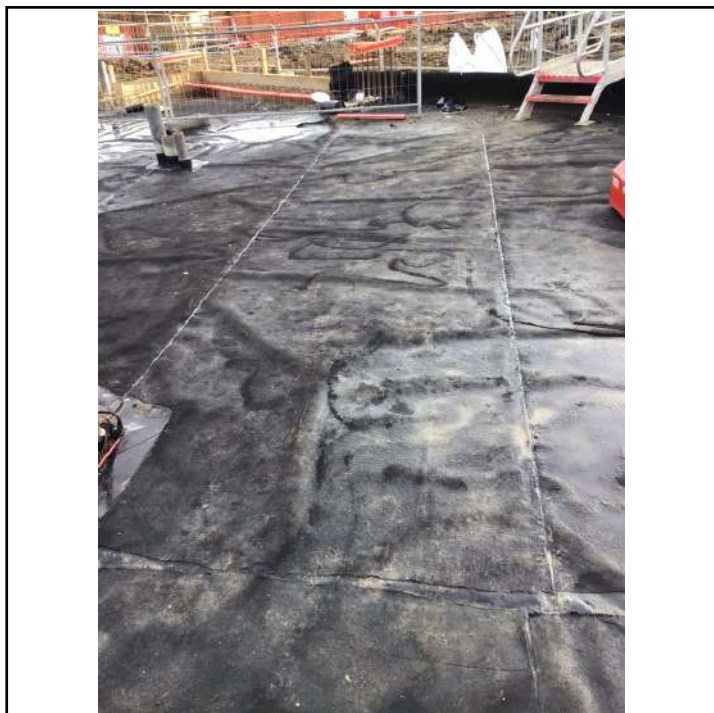
Example of two welded joints air lance tested.
