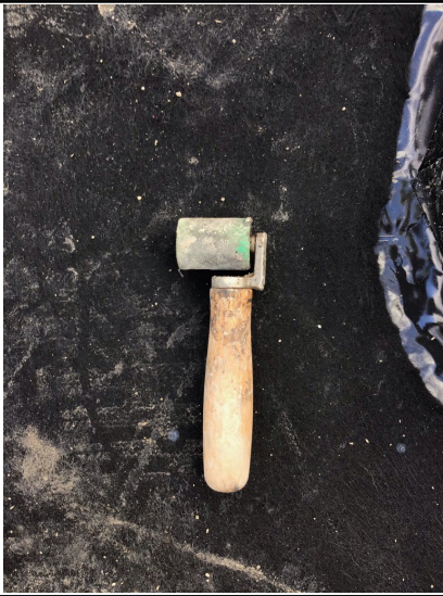
Roller used during install
