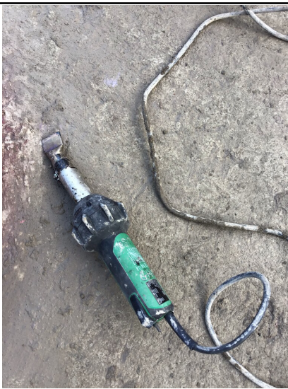
Leister used during install
