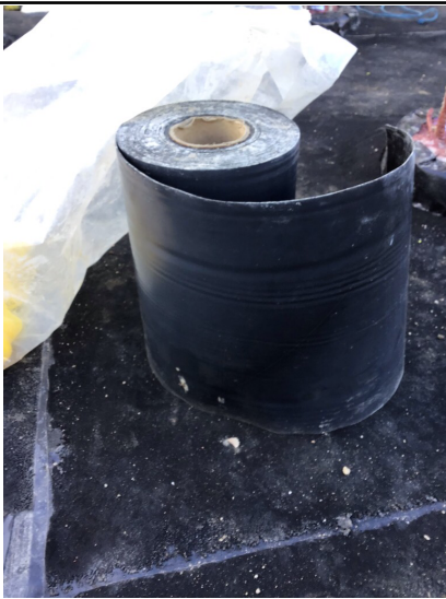
Pudlo jointing tape used on joints and
