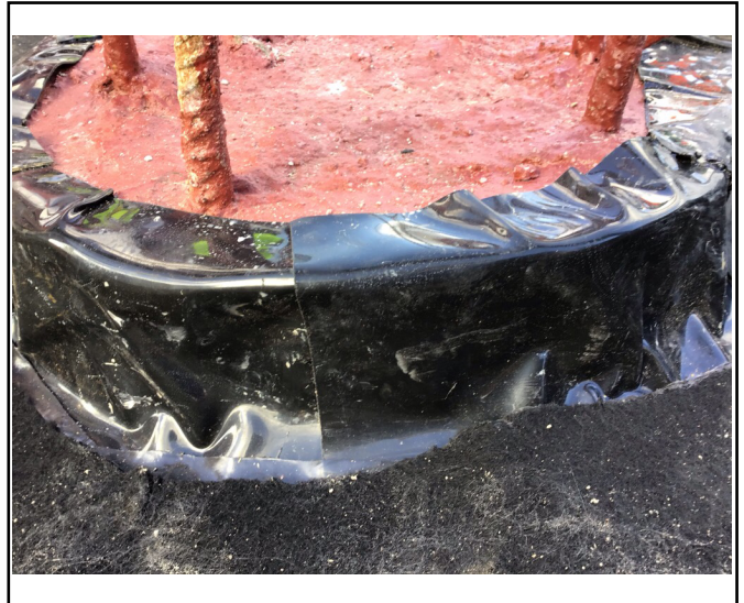
Pile head fully sealed
