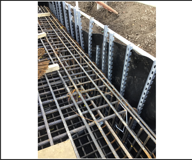
Tric trac spacers to vertical
