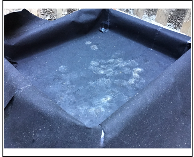
Pump chamber base tested with
