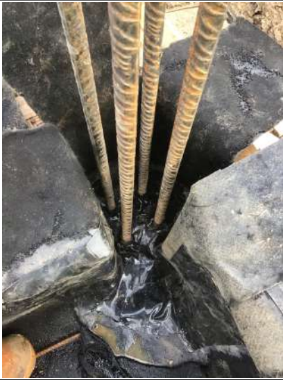
Sealed corner detail.
