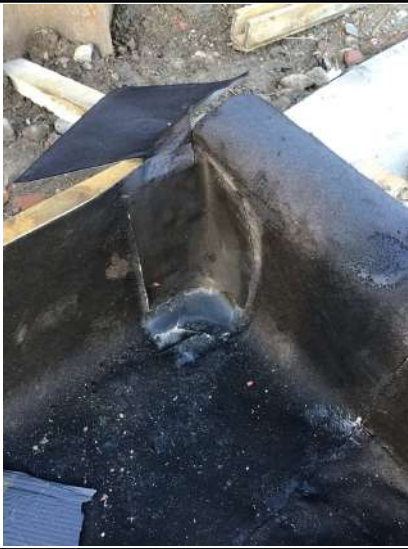
Sealed corner detail using EXT tape.
