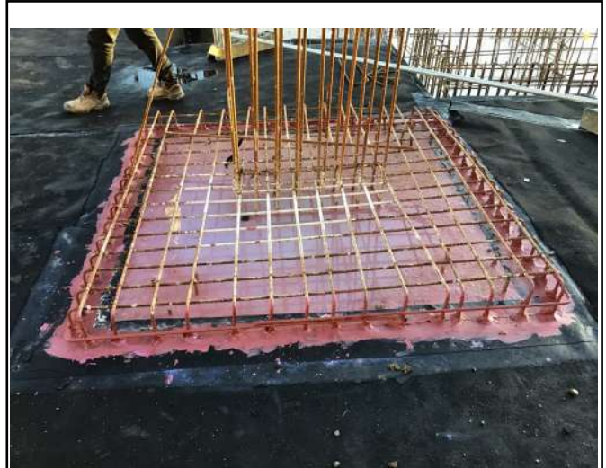
Sealed pile using Pudlo liquid
