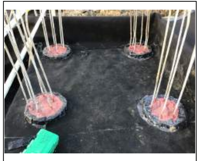
Additional sealed pile caps.
