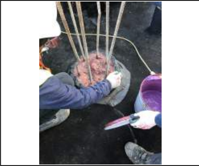
Installers applying the Pudlo Liquid
