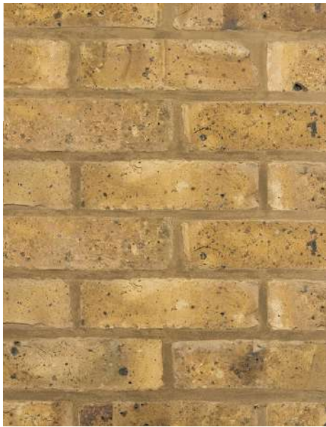
(9) Existing dwarf garden wall
