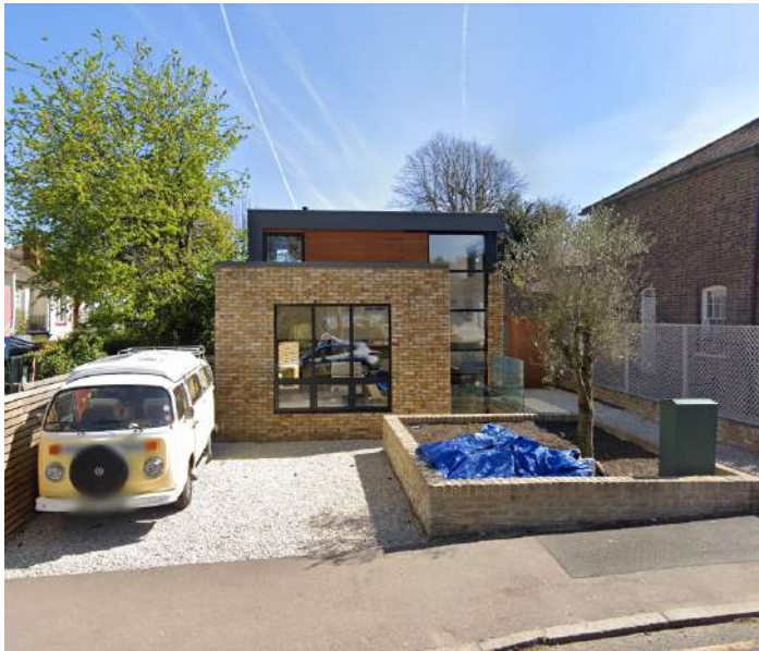
Latest observed condition on site, dwelling close to completion
