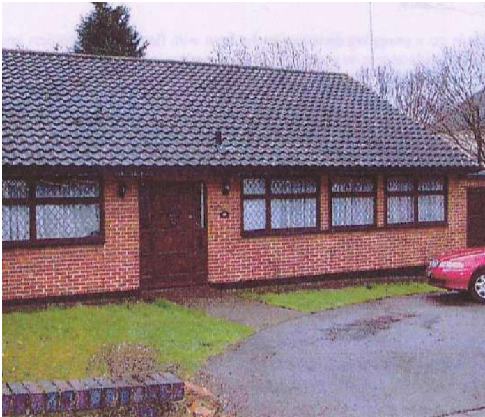
Original Dwelling - No.35A Wood Vale
