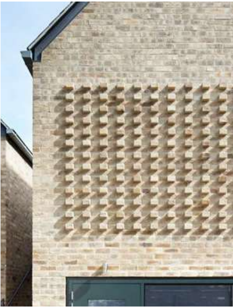
(2) 'Hit and miss' protruding brickwork
