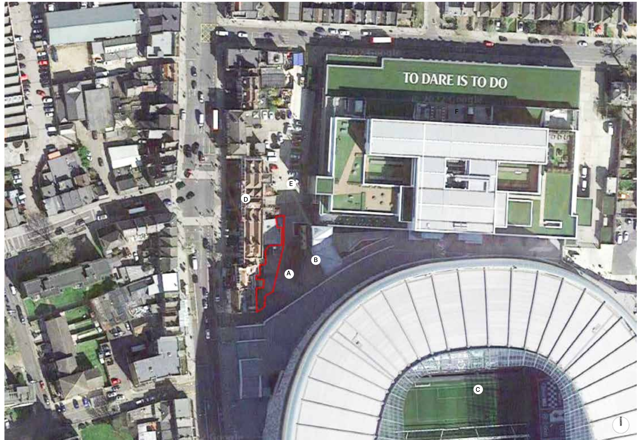
FIGURE 8. Site Aerial View
