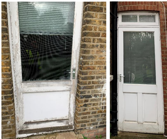
Figure 3: : Existing rear doors
