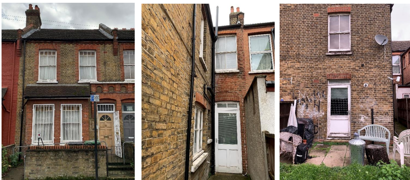
Figure 1: Existing windows on the building
