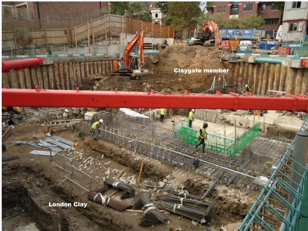
Photo 4 Basement trench, looking southwest
