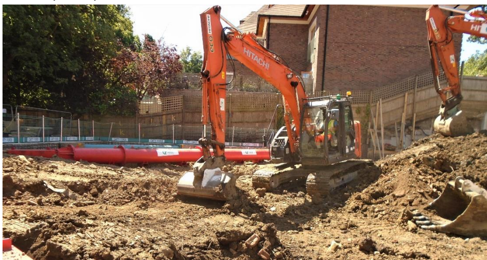
Photo 1 Main excavations, looking south
