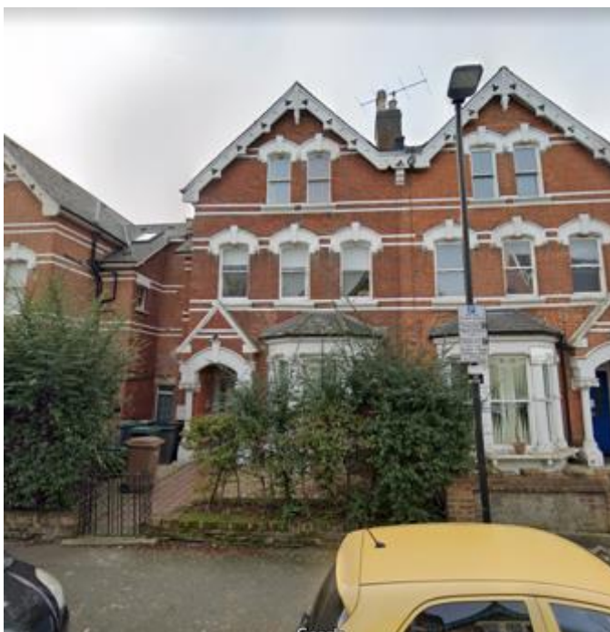
Front elevation of main property
