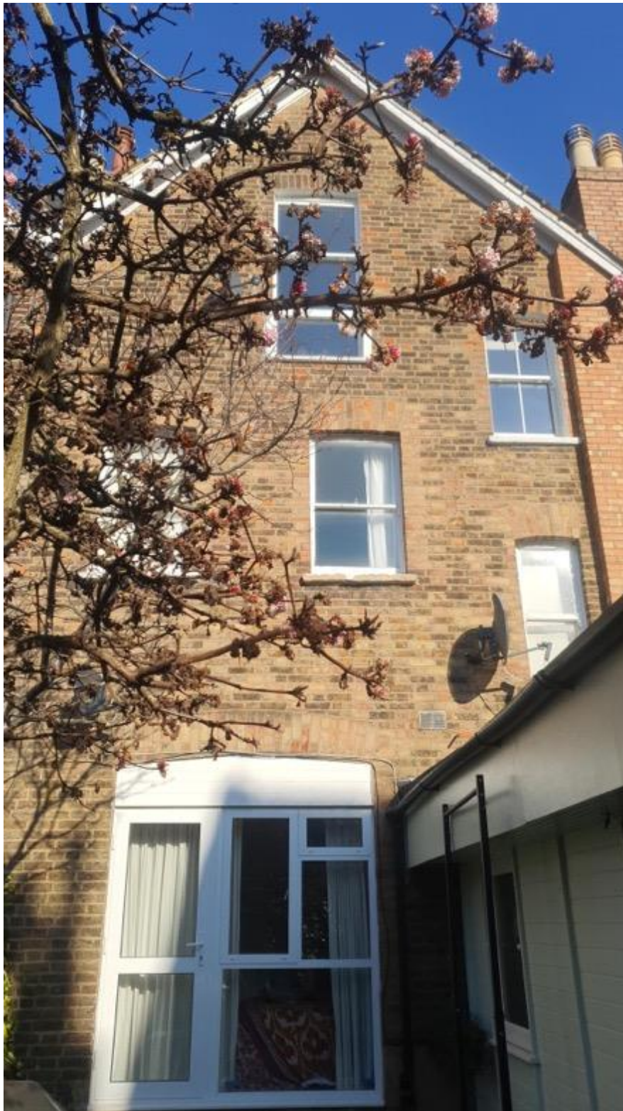
Rear elevation of main house
