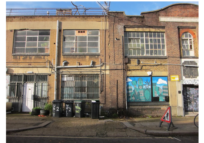
Infill facade block from the 1950s (left), historic facade (right)
