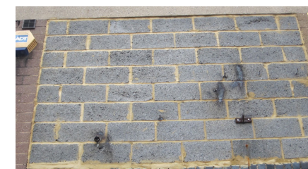
③A Example of material to be broken down for foundations or hard landscaping
