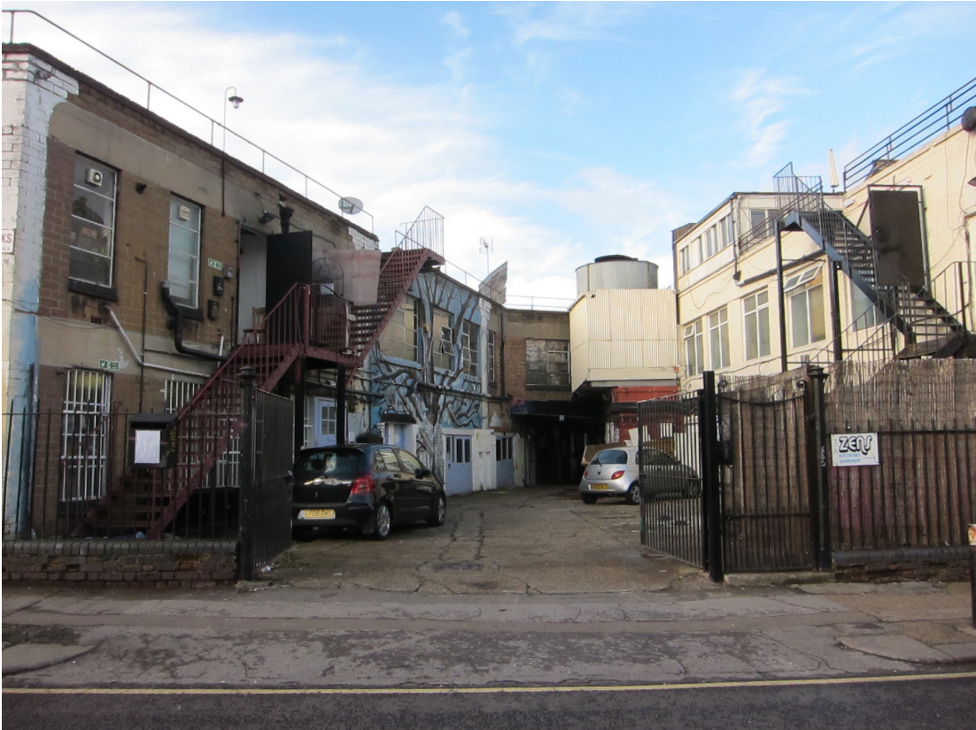
View of external space seen from Hermitage Road west entrance
