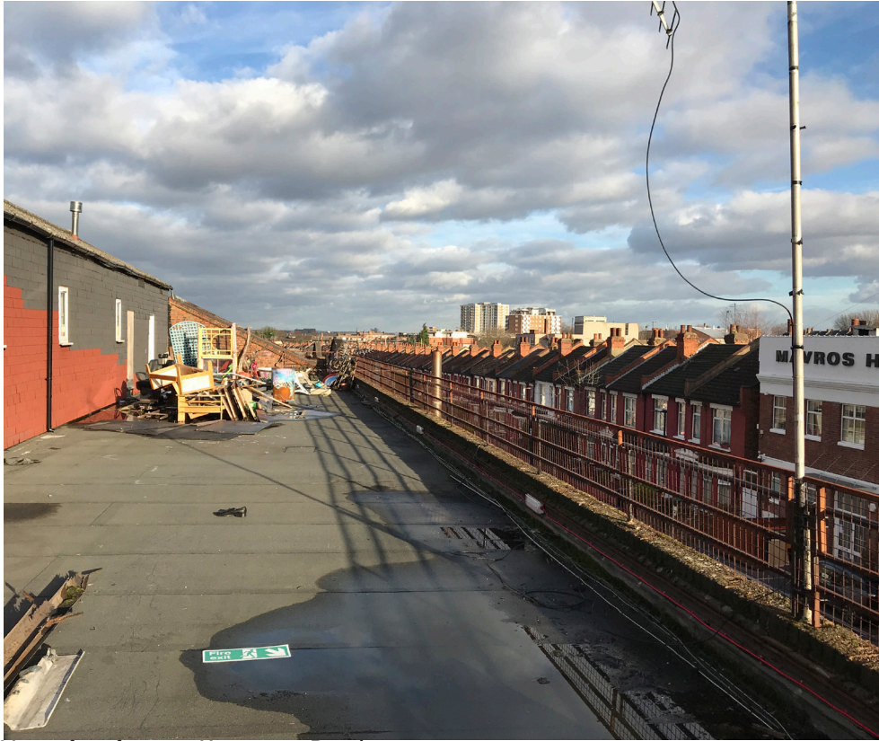
View of roof top on Hermitage Road
