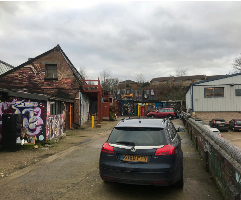
View of rear of site facing west, with Crusader Estate on the right
