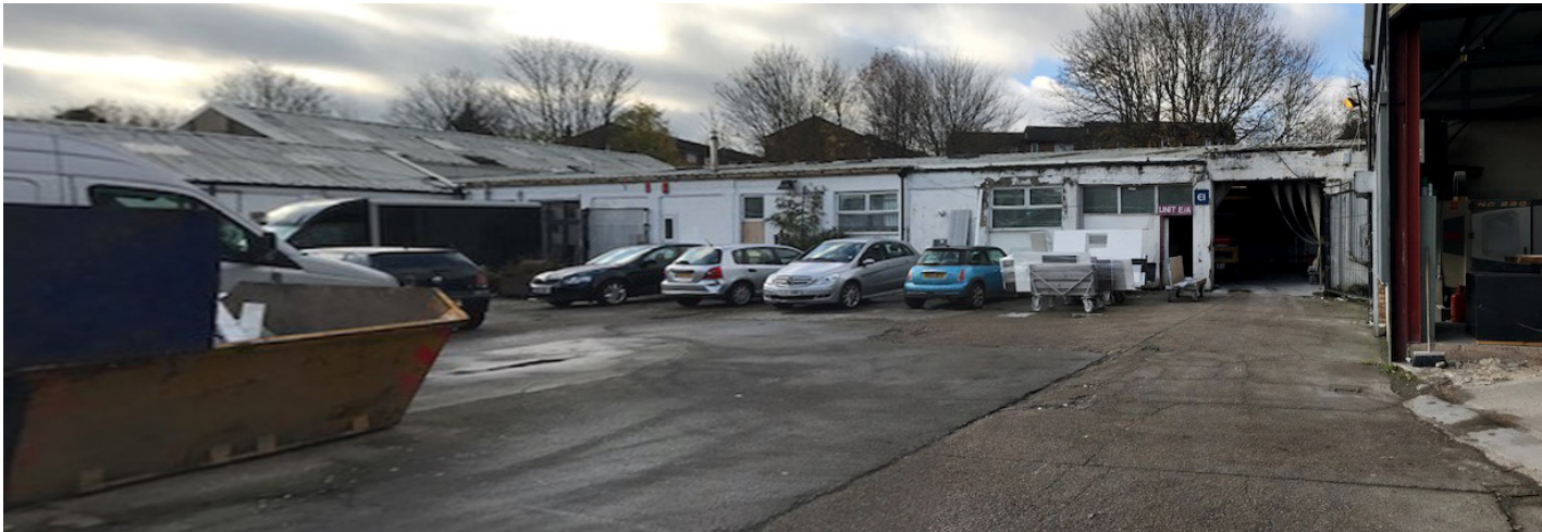
Arena Design Centre: Existing Elevation of Unit E Right facing the communal courtyard
