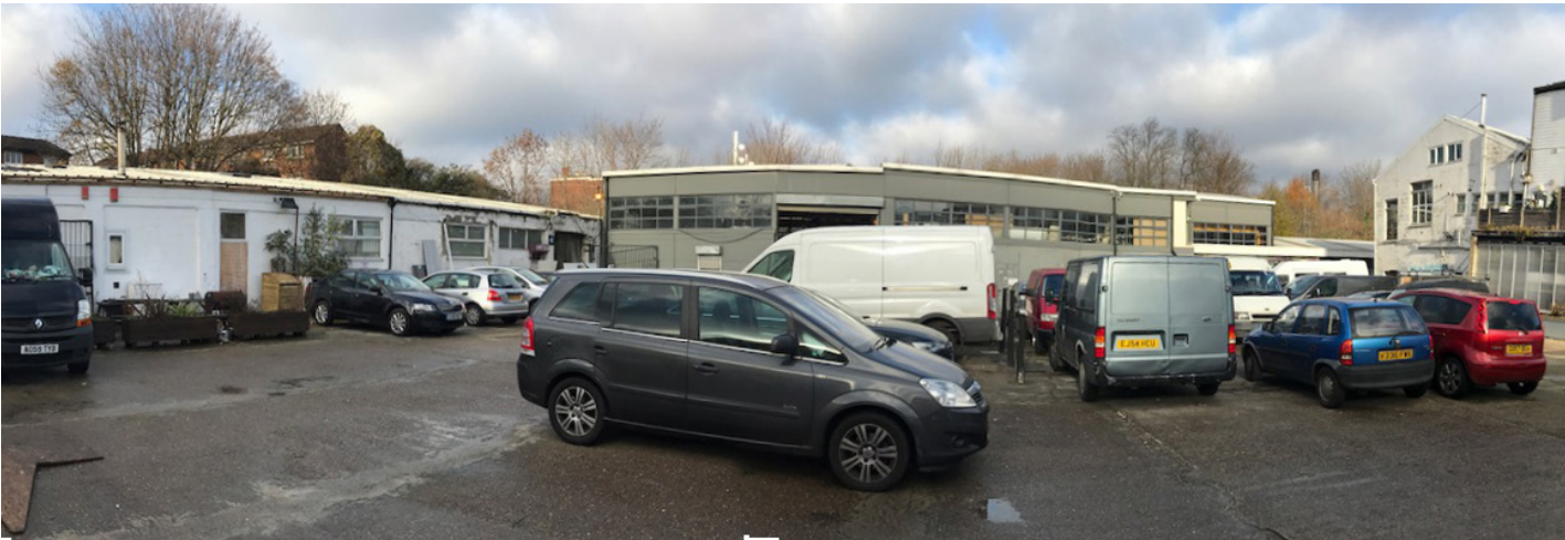
Arena Design Centre: Existing Elevation of Unit D and E Right facing the communal courtyard
