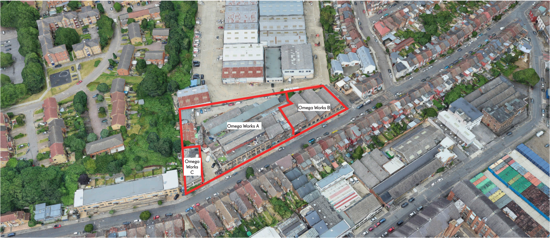
Aerial view with application site labelled 'Omega Works A'
