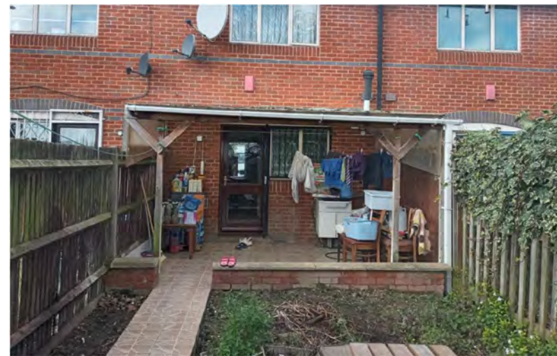
Figure 6.3: Photograph of rear of 78 Finsbury Park Avenue showing ground floor canopy
