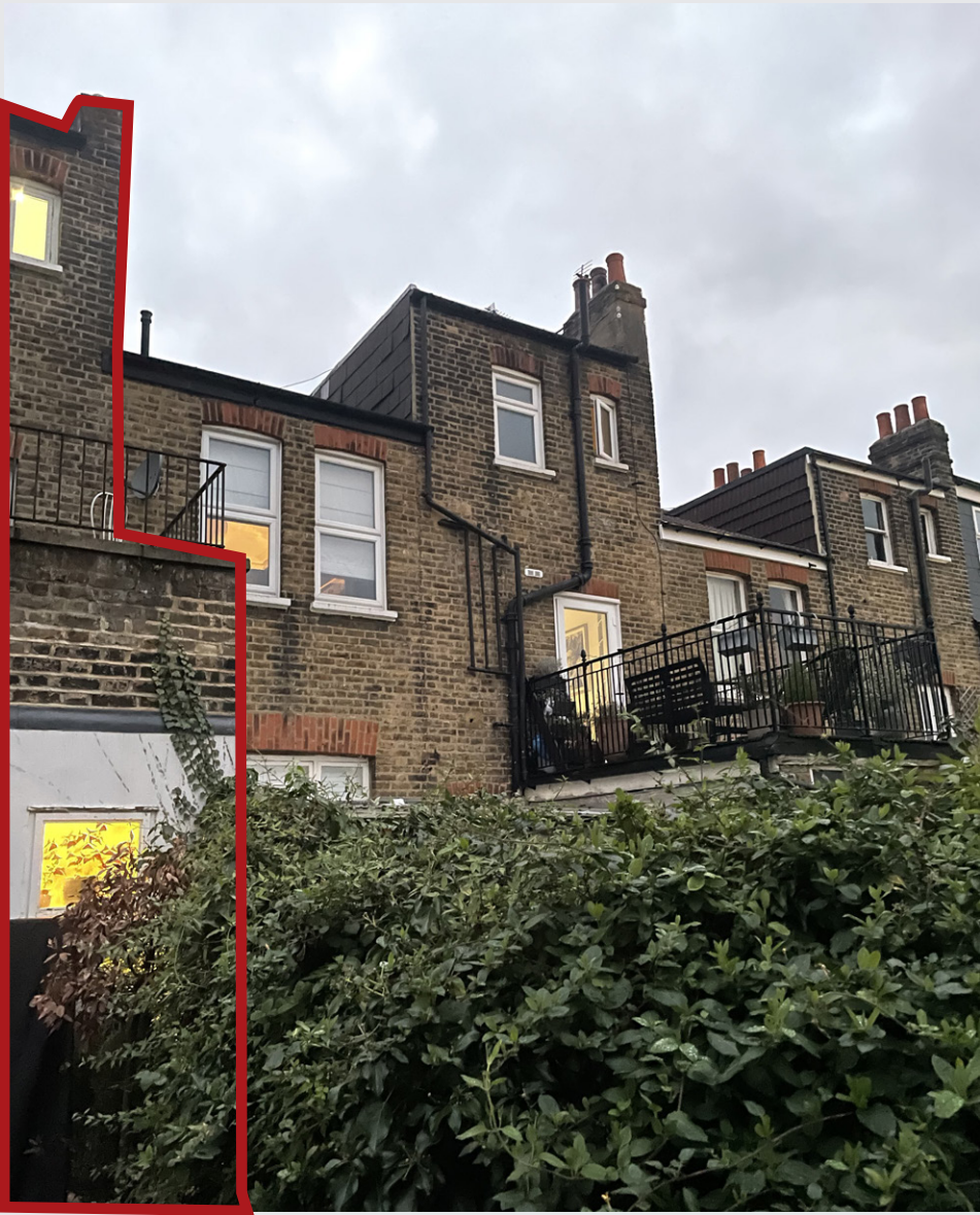
Rear Elevation looking north
