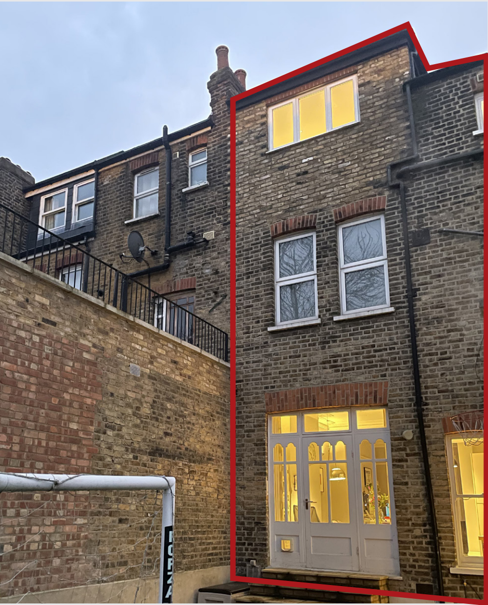
Rear Elevation looking south
