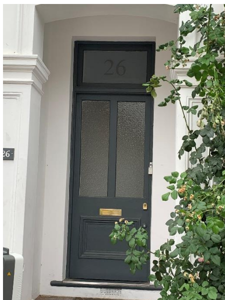
Figure 4: Existing front door
