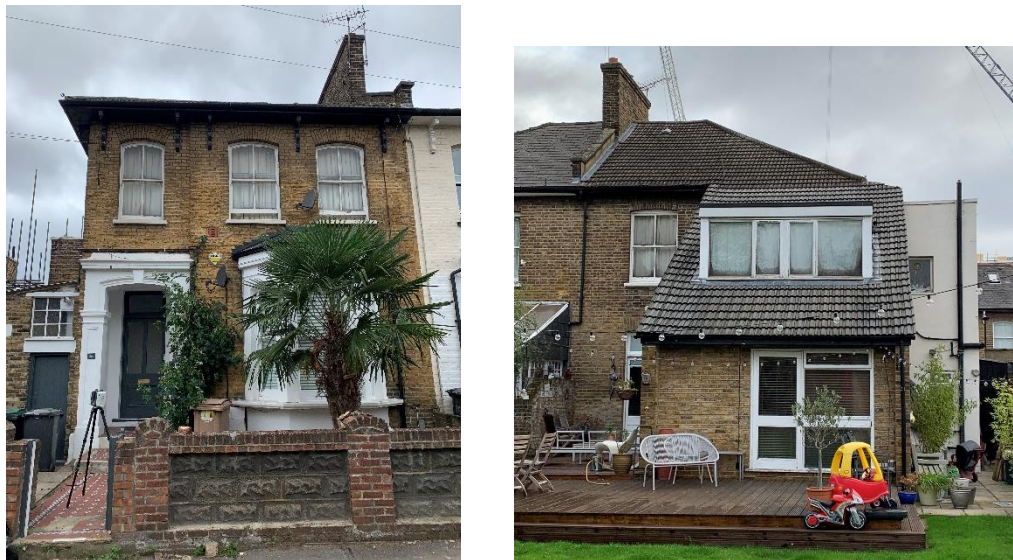
Figure 2: Existing windows on front and rear elevation
