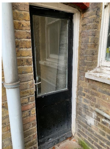
Figure 4: Existing rear door
