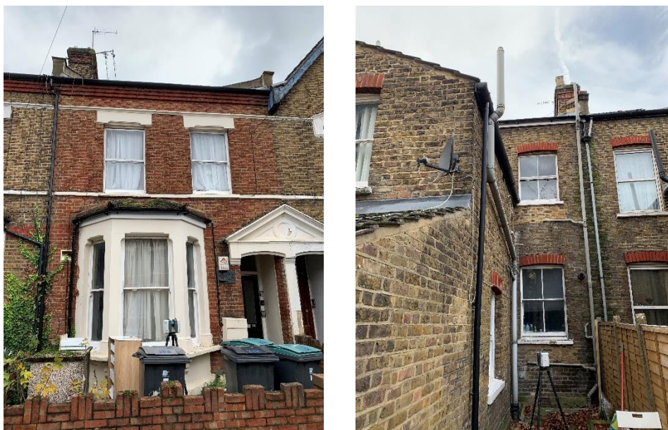
Figure 2: Existing windows on the building
