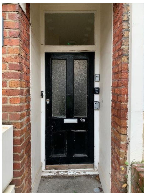
Figure 3: Existing front entrance door
