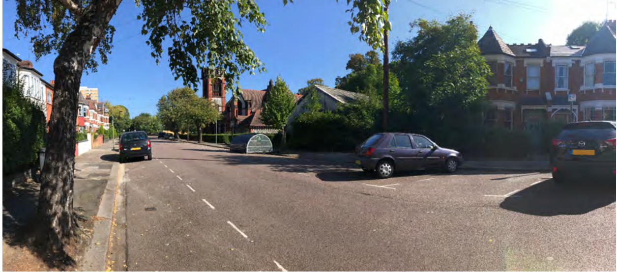
Photograph of existing church and properties in Braemar Avenue
