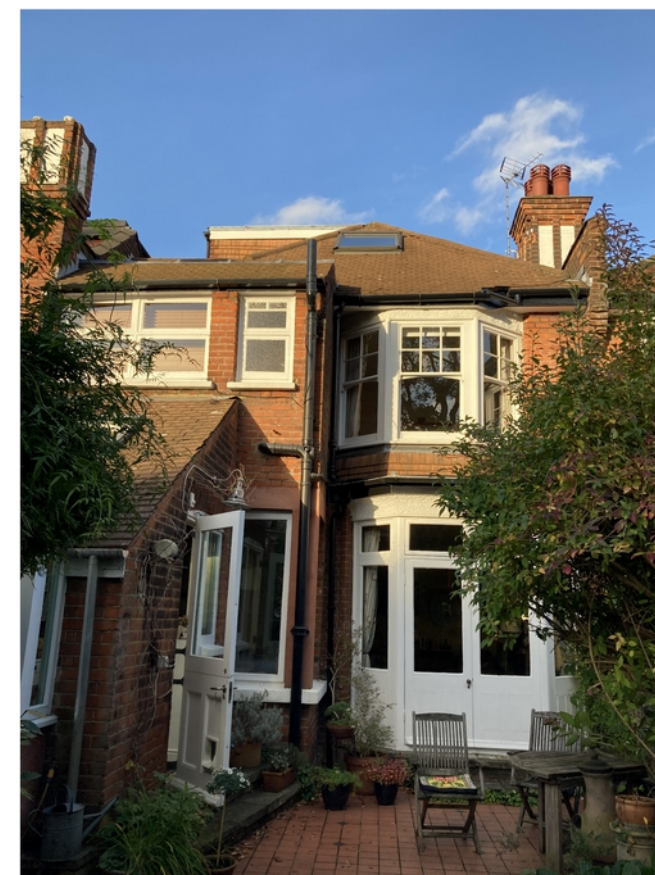
19 Woodberry Crescent with existing roof light
