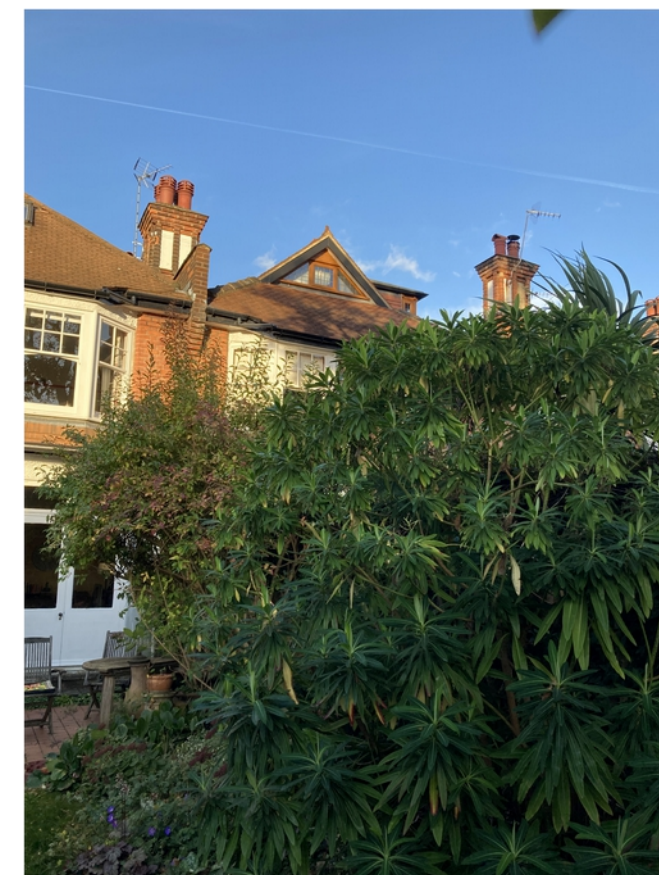
17 Woodberry Crescent, with dormer
