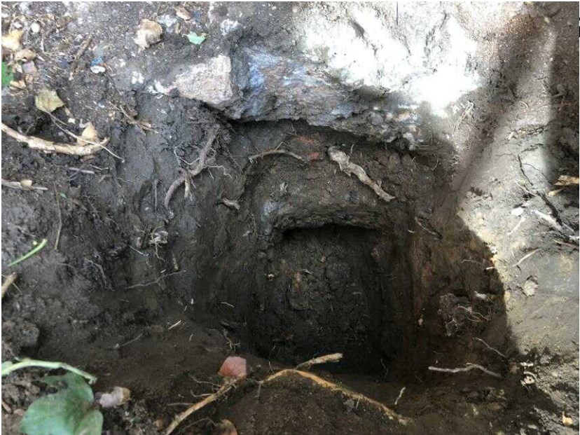
FP04 View of Exposed Foundations
