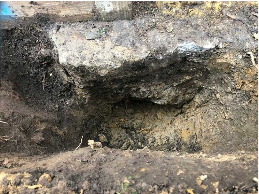
FP02 View of Exposed Foundations
