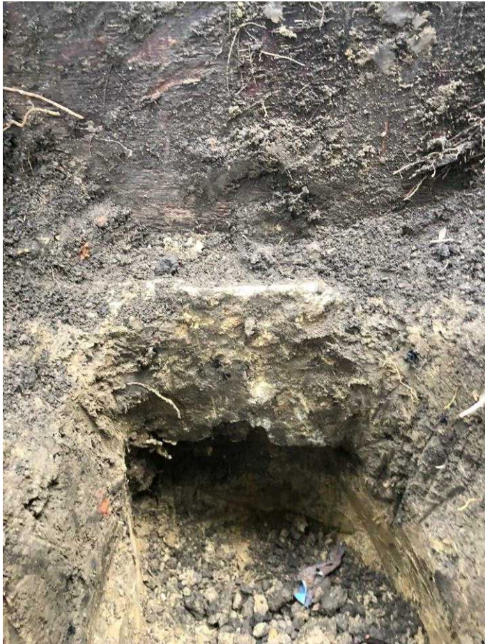
FP03 View of base of Foundations
