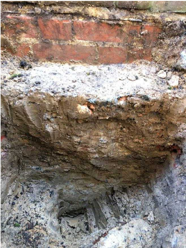
FP01 View of Exposed Foundations
