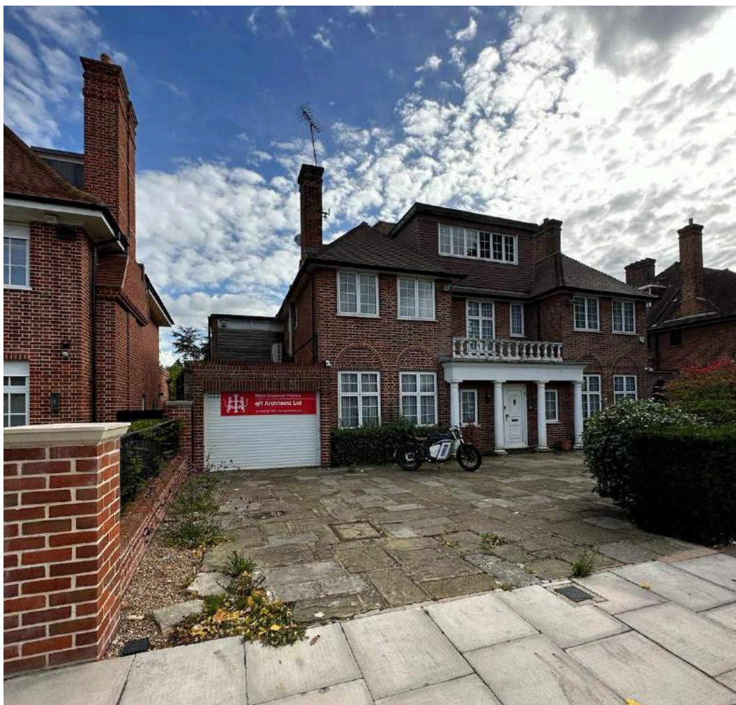
No.26 Sheldon Avenue - Boundary with no.28
