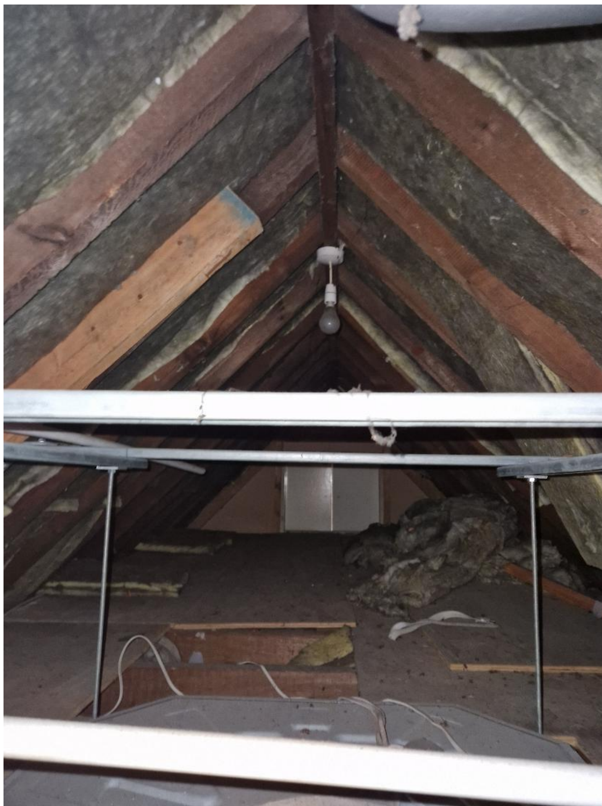
Plate 7: Photograph displaying the roof interior of the surveyed structure.
