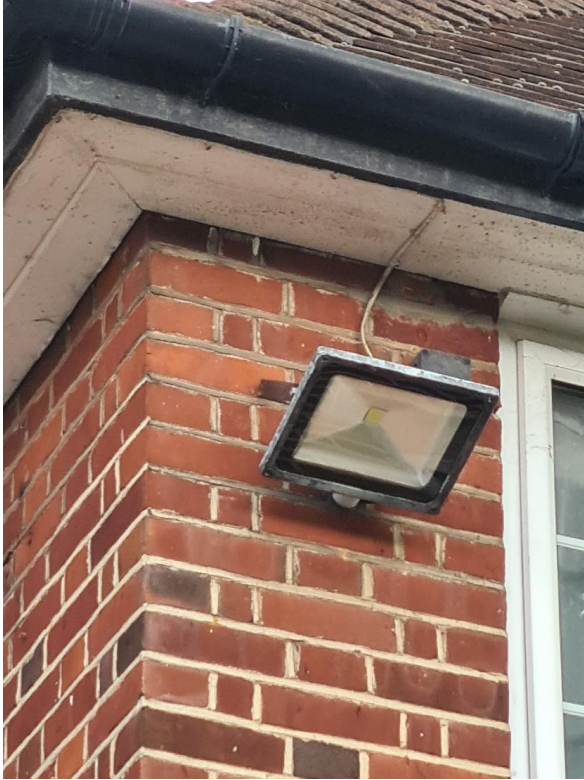
Plate 6: Photograph displaying gaps underneath the eaves, providing potential access for bats.
