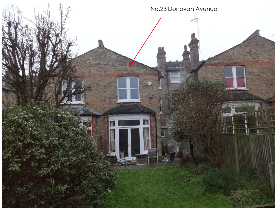
Figure 1.2 Existing rear elevation
