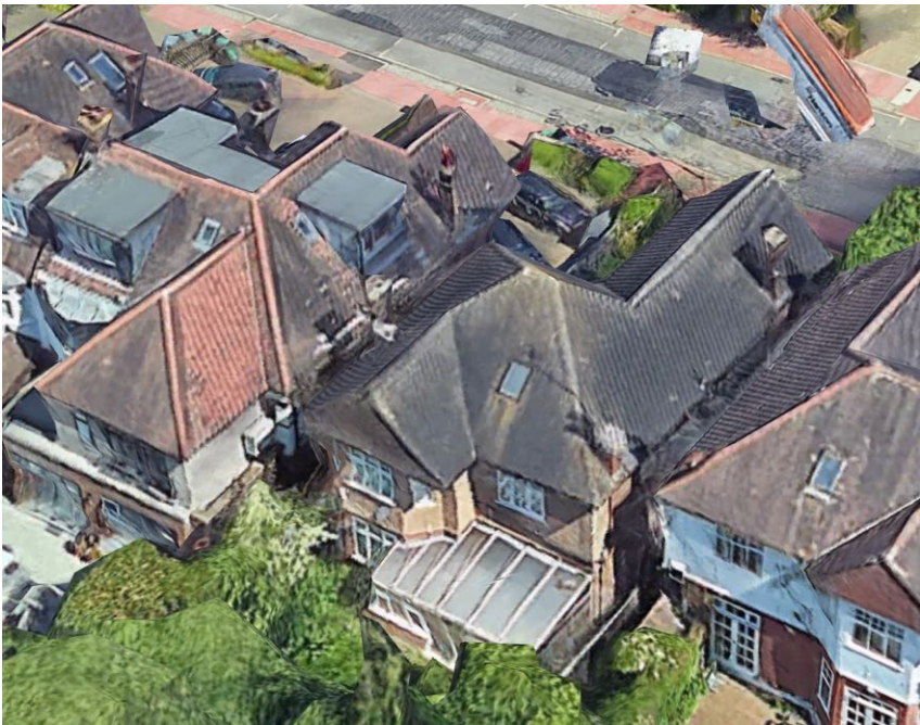
AERIAL PHOTO OF 23 BANCROFT AVENUE AND NEIGHBOURING NUMBER 25 WITH REAR EXTENSION
