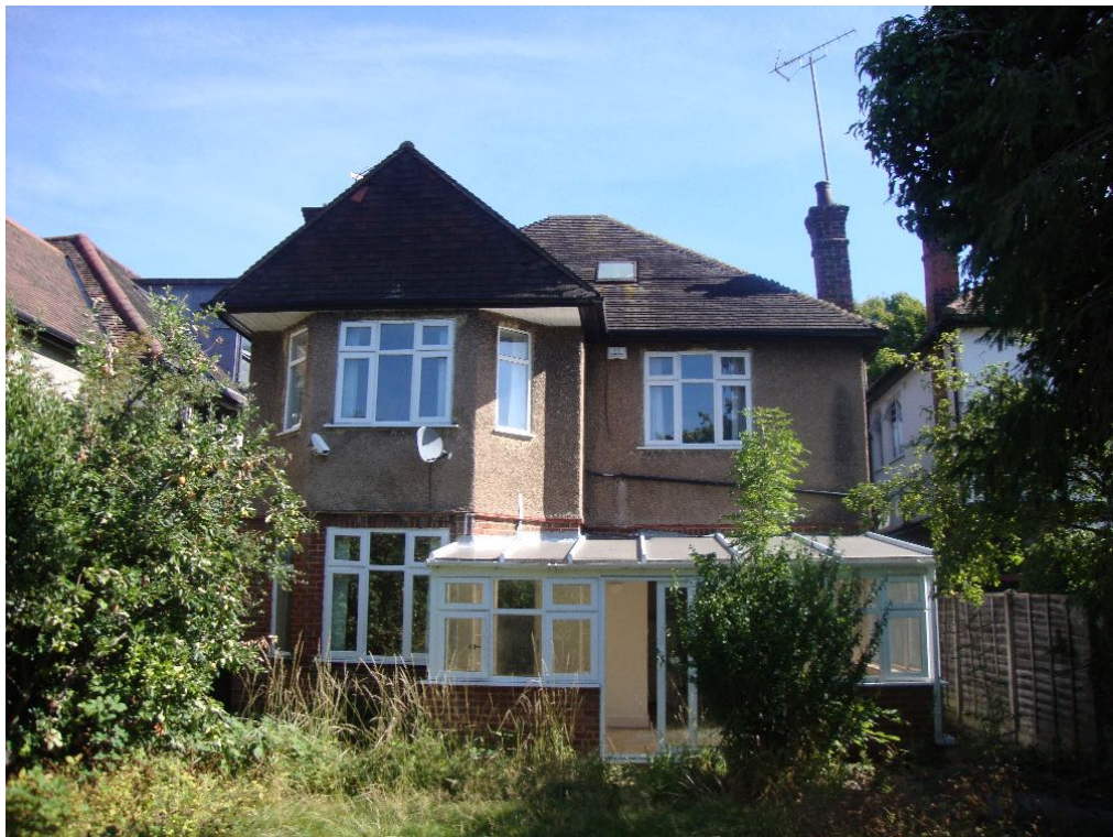
REAR ELEVATION OF 23 BANCROFT AVENUE TAKEN FROM THE REAR GARDEN
