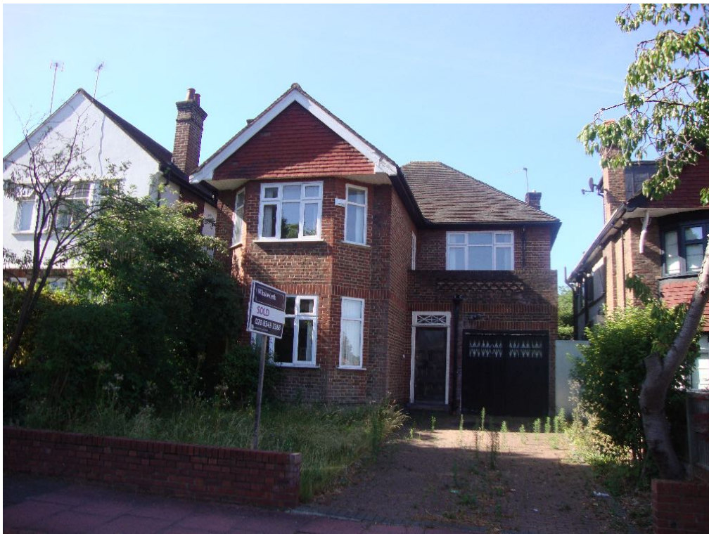
FRONT ELEVATION OF 23 BANCROFT AVENUE TAKEN FROM THE STREET
