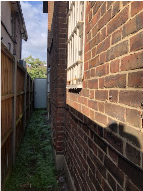
RHS ELEVATION OF 23 BANCROFT AVENUE LOOKING TOWARDS THE FRONT OF THE PROPERTY. TAKEN FROM SIDE PASSAGE
