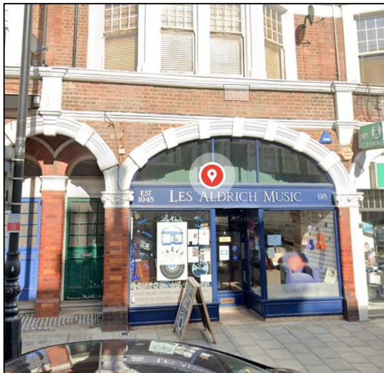
Figure 1 – Front Elevation of No. 98 Fortis Green Road.
