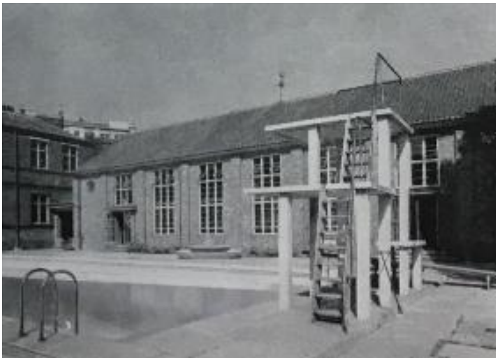
Figure 30. Completed swimming pool seen looking north.
