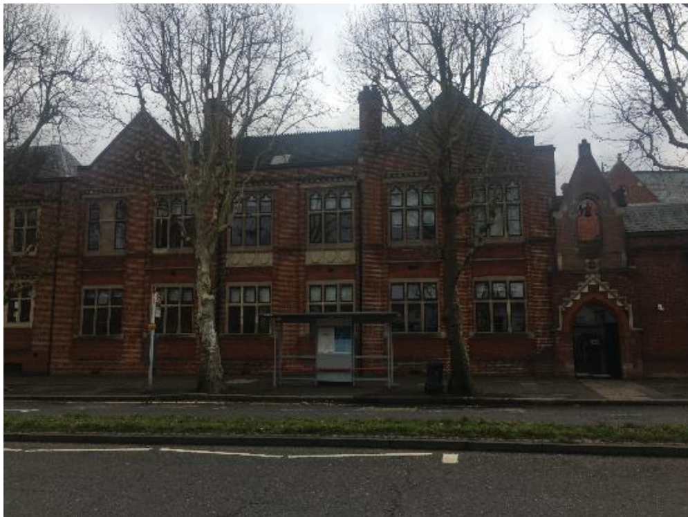
Figure 74. View of Central Hall western façade seen from North Road to the west. Note decorative treatment to the fenestration in comparison to the rear Science Quad elevations.
