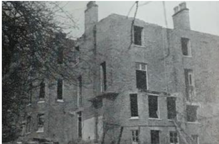
Figure 36. Demolition of the old Dyne House.
