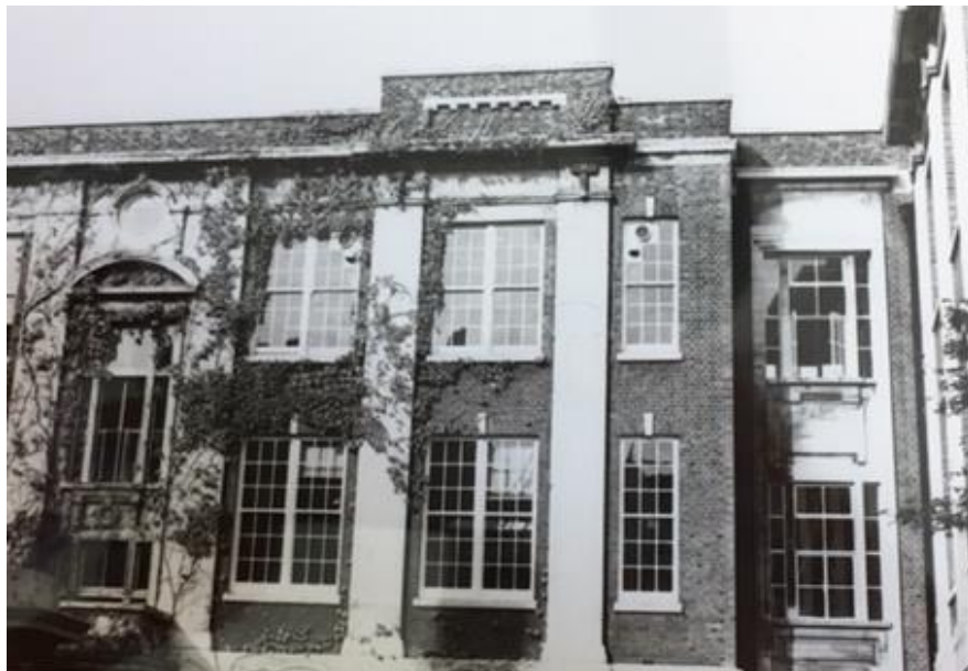
Figure 23. View within Science Building Courtyard, circa 1940s. Note change in fenestration within entrance bay to the right of the image and above entrance bay to the left.
