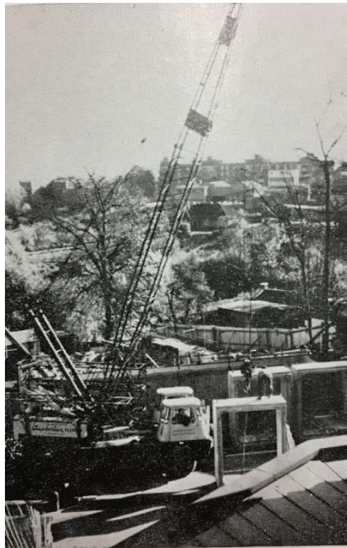
Figure 38. Instillation of the tunnel to Dyne House.
