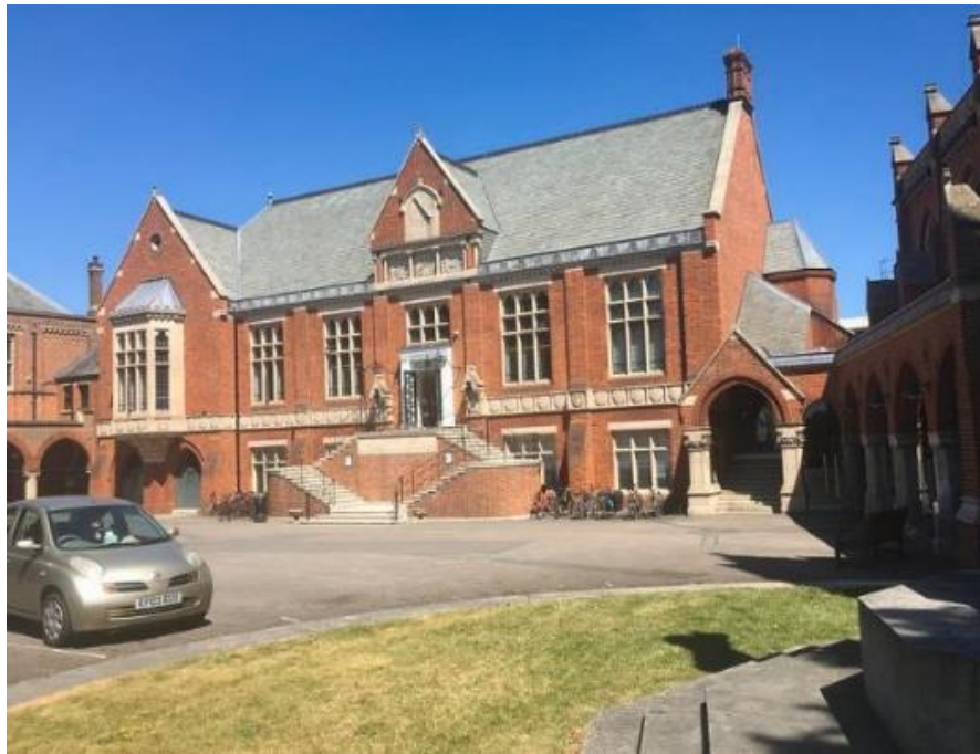
Figure 91. 'Big School' or the 'Old School Building' Grade II, to the south of the site seen from North Road. The Chapel is visible to the right and the 1890s extension just visible to the left. The steps are a later addition, added as a memorial post 1945.
