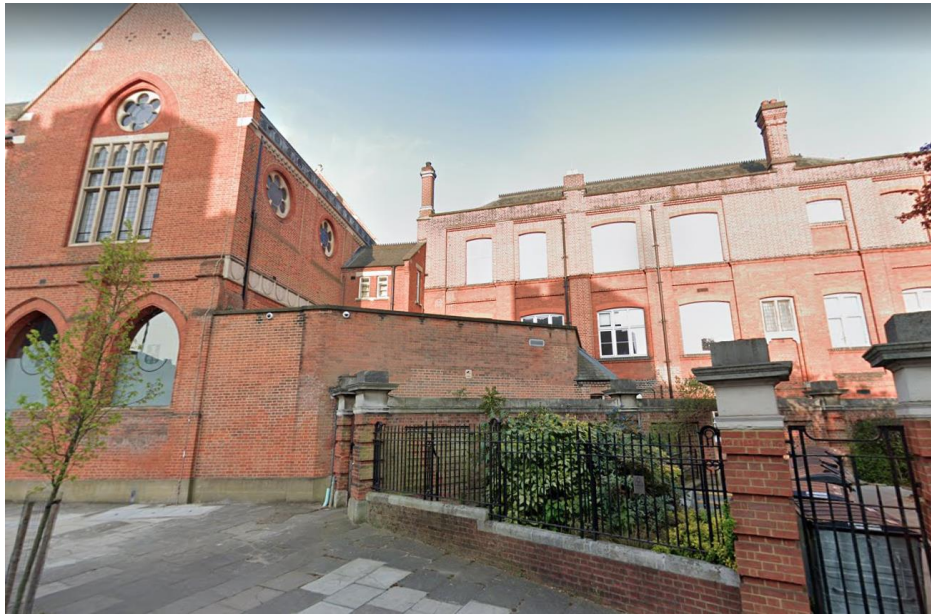
Figure 72. View of eastern façade of the Central Hall and Science Quad. Note the plain appearance of the toilet block adjacent to the eastern façade of the hall.
