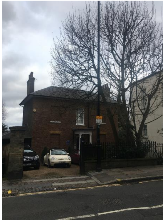
Figure 97. 22 Southwood Lane, views from the west.
