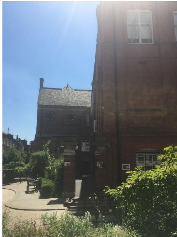
Figure 79. View south from the Science Quad looking towards the single storey brick structure housing WCs and ancillary services adjacent to the eastern façade of the Central Hall.
