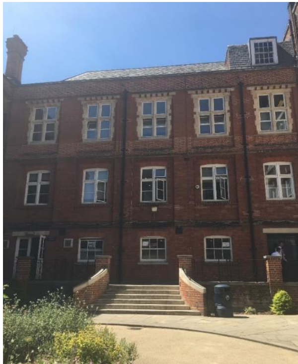
Figure 83. Northern elevation of nineteenth century Central Hall block opposite the Science Building.
