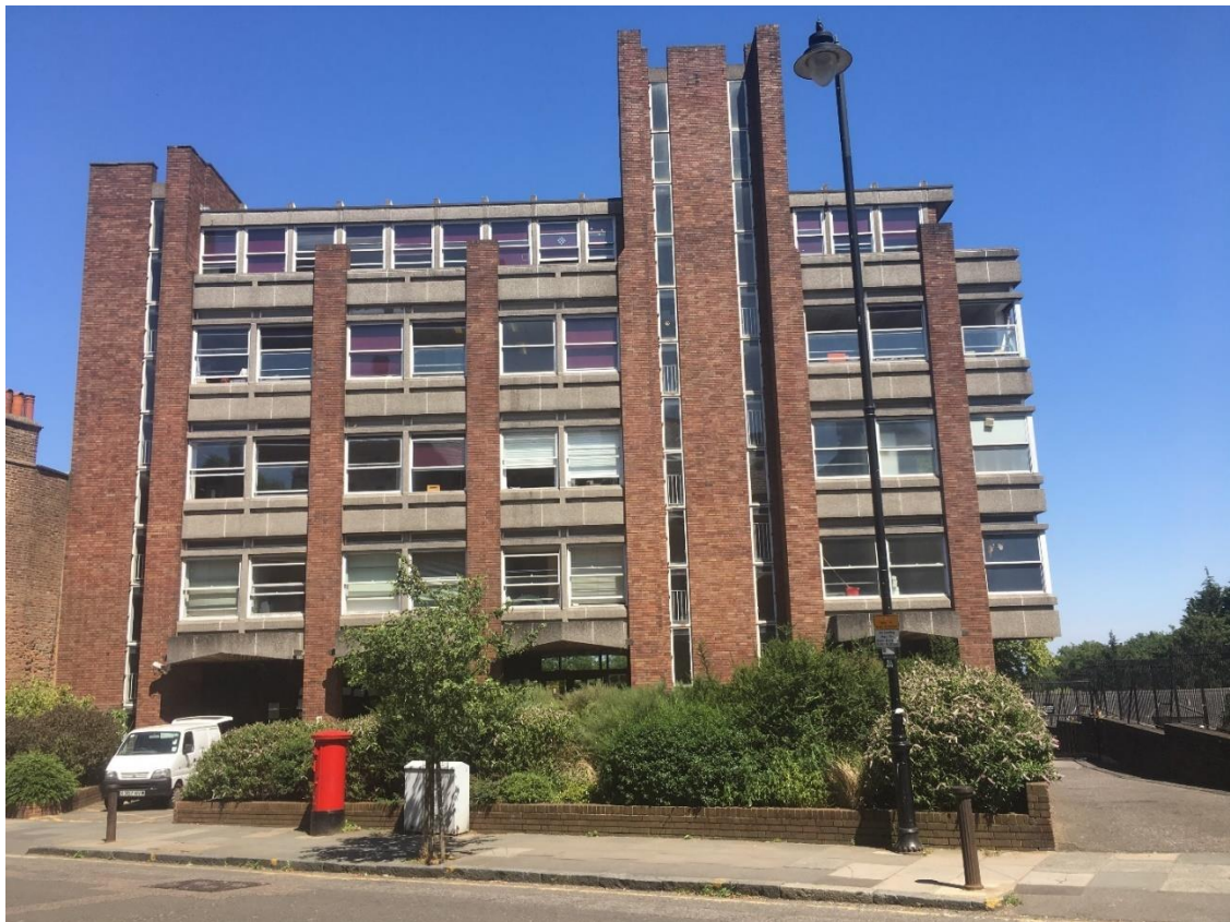
Figure 57. View of Dyne House seen from the west on Southwood Lane.
