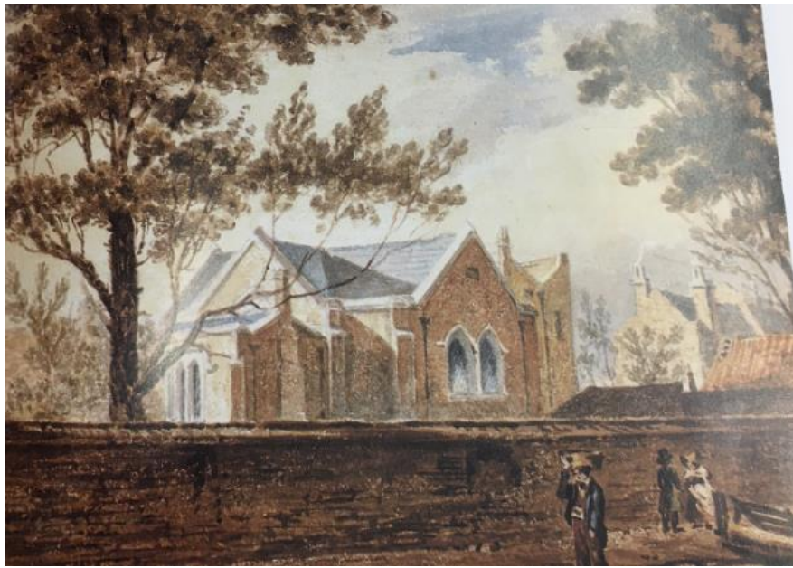
Figure 9. The Old School in 1833 viewed from Southwood Lane following the demolition of the chapel and prior to the extension works of 1845.
