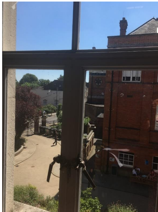
Figure 80. View south from the Science Building towards the single storey link building between the Central Hall and Big School adjacent to the eastern façade of the Central Hall.
