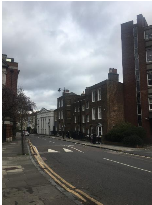
Figure 95. View of 16-22 Southwood Lane from the south.
