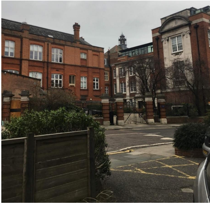
Figure 77. View of the Science Quad from Dyne House, note the single storey brick infill block between the Central Hall and big school blocks views of the eastern façade of the building.
