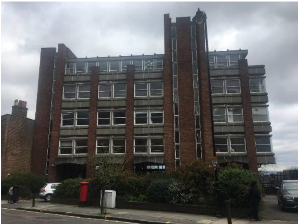
Figure 39. View of Dyne House seen from the west on Southwood Lane.
