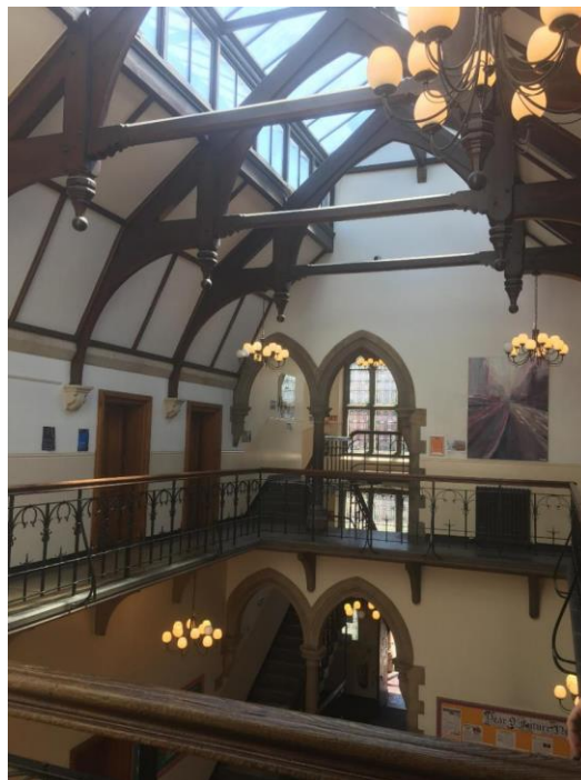
Figure 85. Central Hall, note gothic detailing including pointed arches, stone mullions to windows and tri-foil ironmongery to balustrade.
