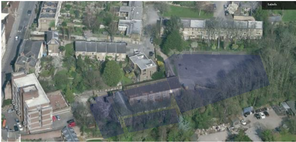
Figure 66. Existing aerial view of the swimming pool, gymnasium complex and parade ground to the east of Dyne House.
