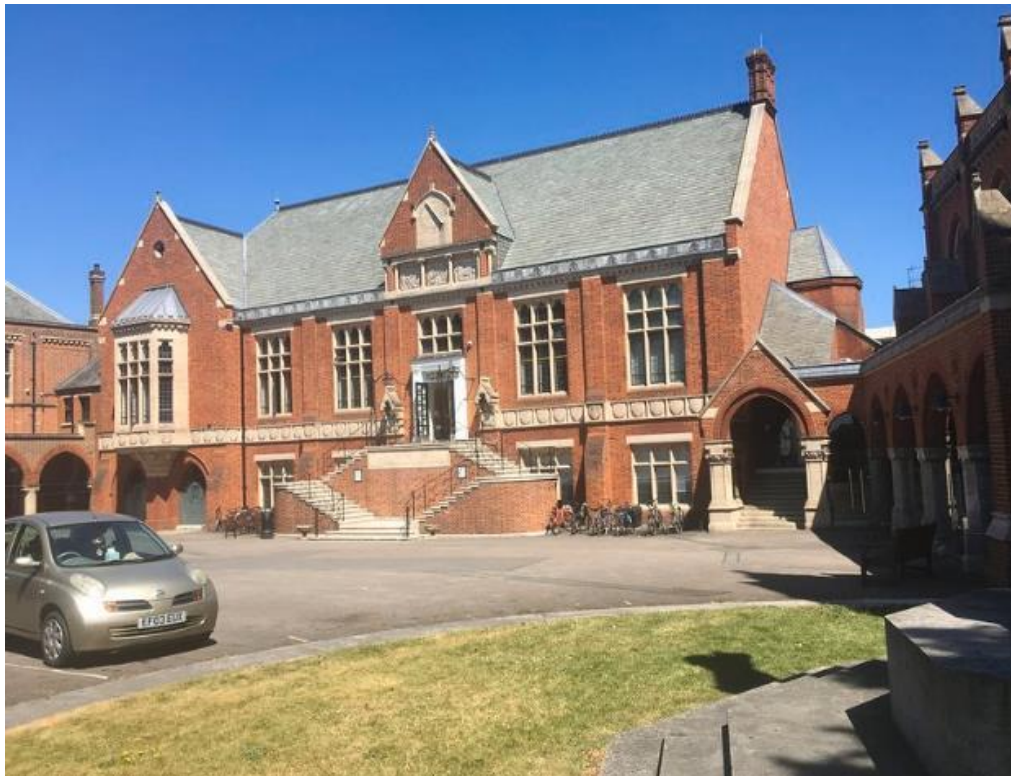
Figure 87. 'Big School' or the 'Old School Building' Grade II, to the south of the site seen from North Road. The Chapel is visible to the right and the 1890s extension just visible to the left. The steps are a later addition, added as a memorial post 1945.
