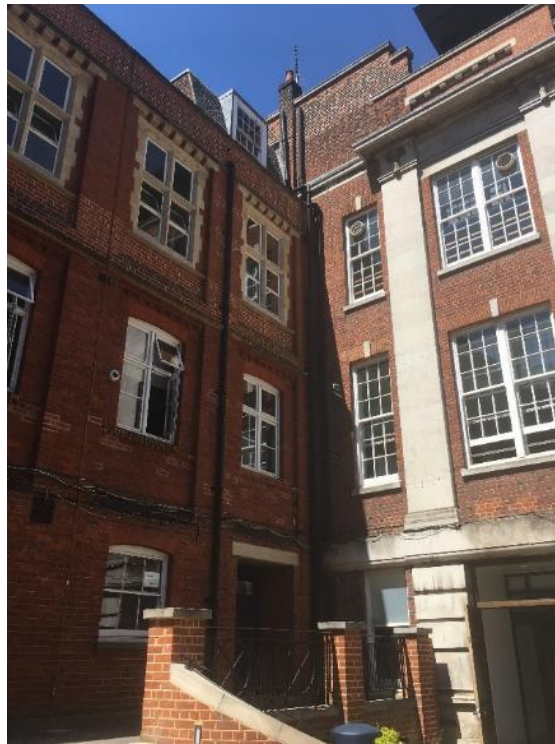
Figure 84. Connection between Central Hall and the Science Building, note modern alterations at ground floor.
