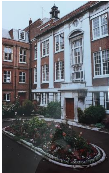
Figure 41. External façade of Science Building Seen from the courtyard, c. 1980.
