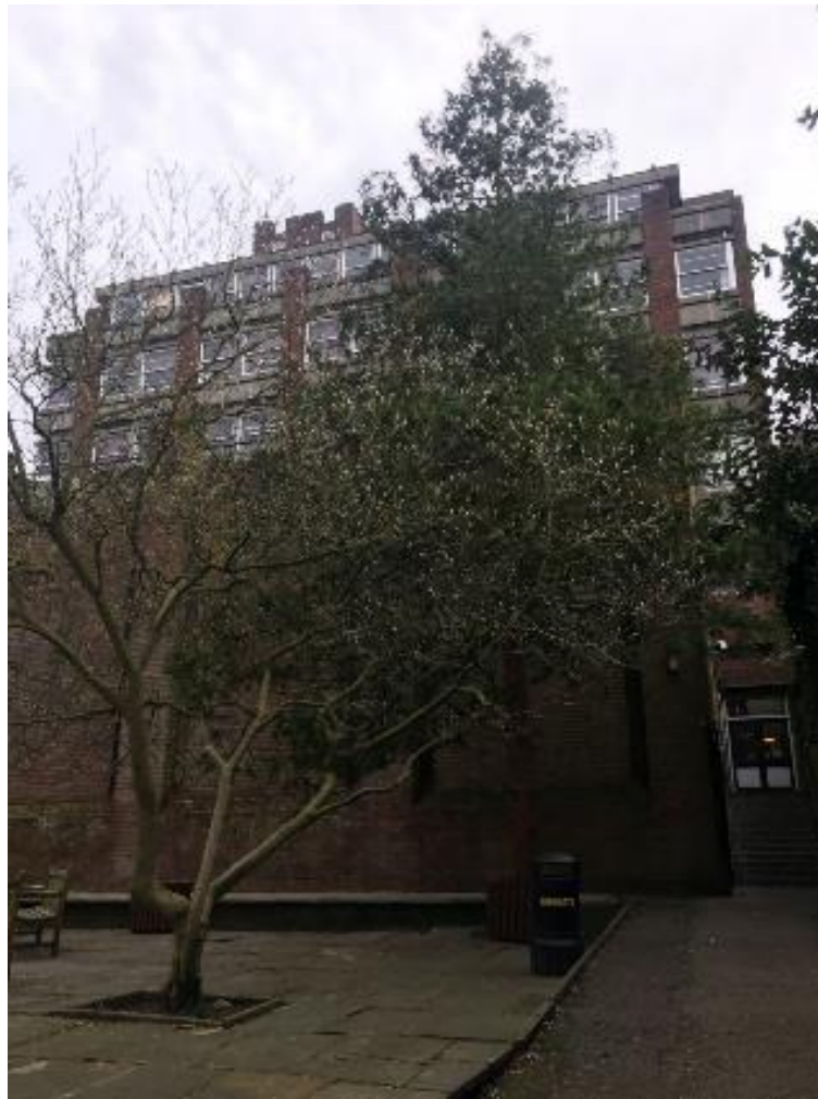
Figure 61. Eastern façade of Dyne House viewed from the east.
