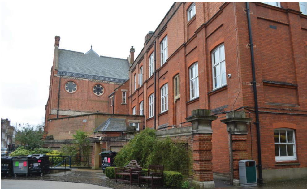
Figure 78. View looking south from entrance into the Science Quad showing single storey brick toilet block building linking the eastern elevation of the Central Hall with the Big School building.
