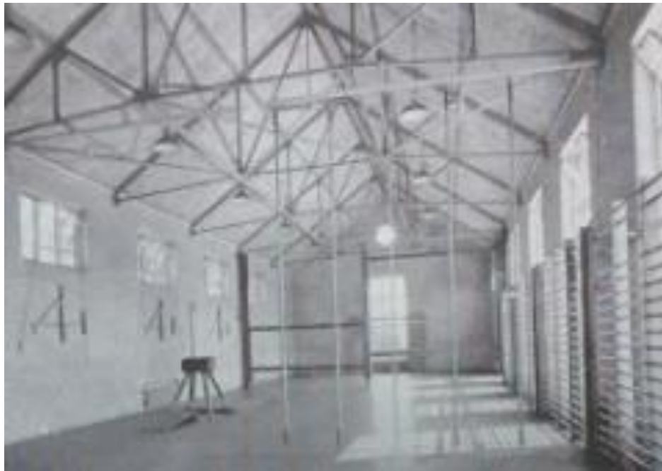
Figure 31. Interior view of the Gymnasium, with metal truss roof structure and timber floor.
