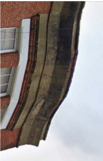
5: Cast stone coping - to match adjacent
