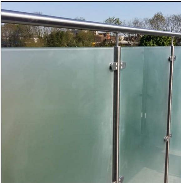
Handrail to Above the Roof Terrace
