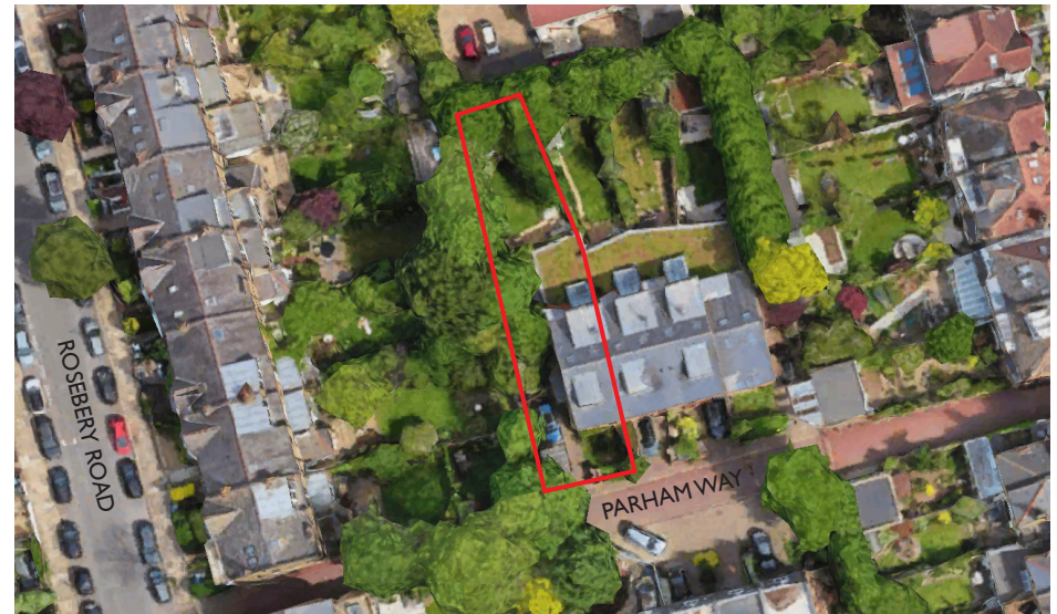
fig 2.2 Satellite view showing site outlined in red
