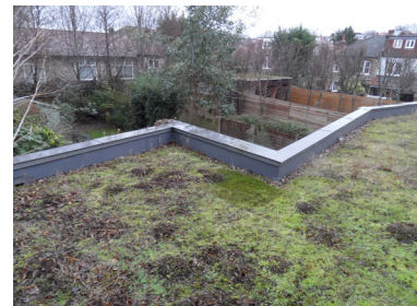
7.9 Green 'living' roof
