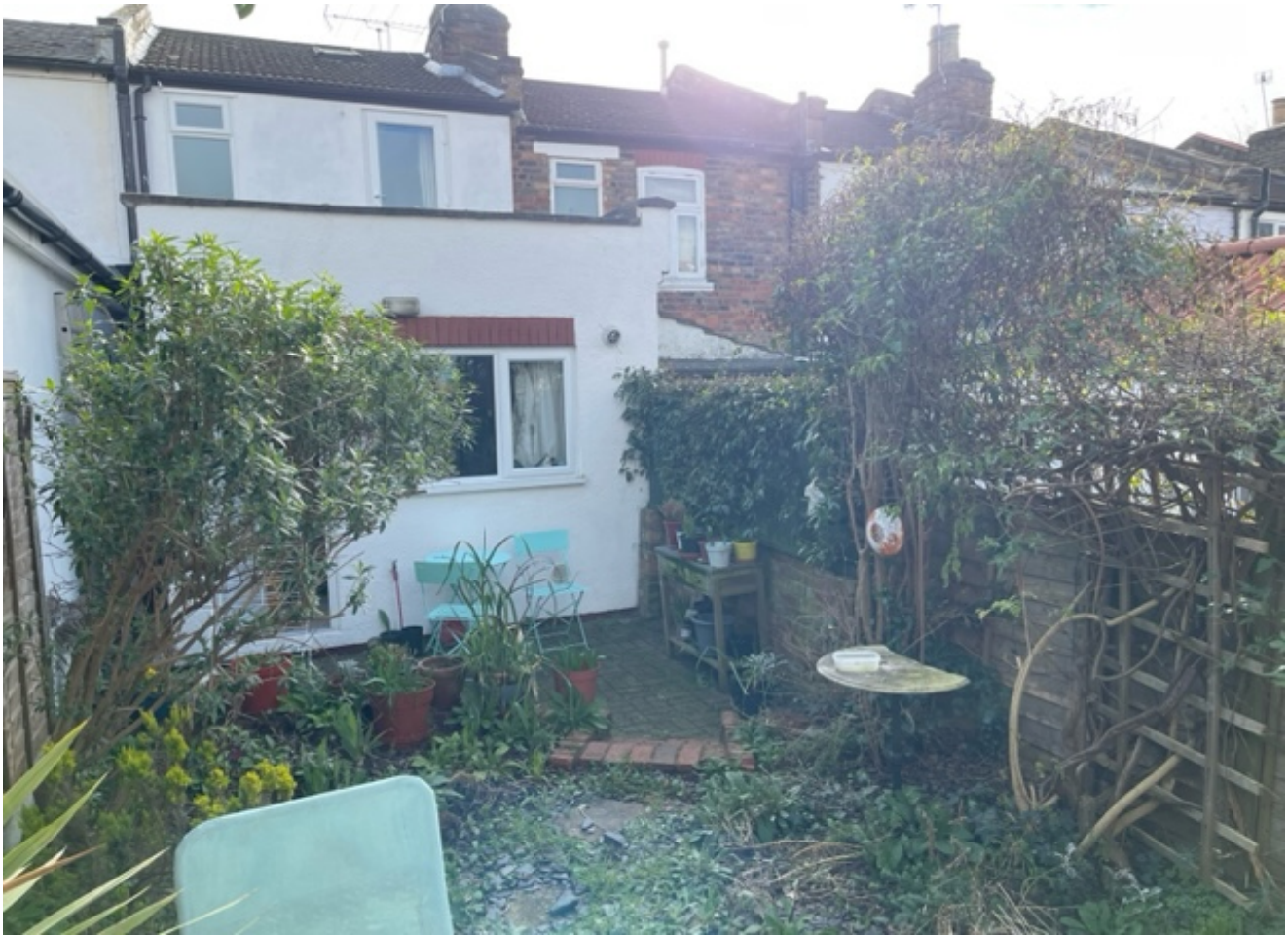
Figure 2 Rear extension of No. 27 in foreground (left side of photograph); No. 25 to right.
